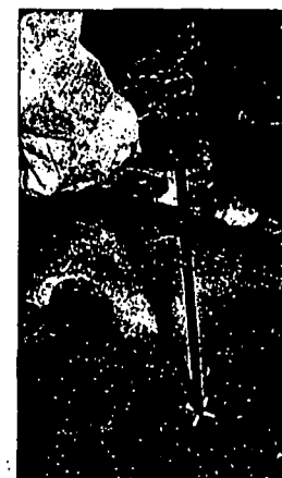
3 Place end of rod on concrete to be pierced for bolts, turn on current
