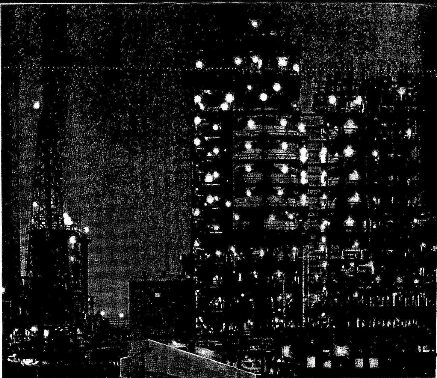
Typical catalytic cracking unit using thousands of Crane products
