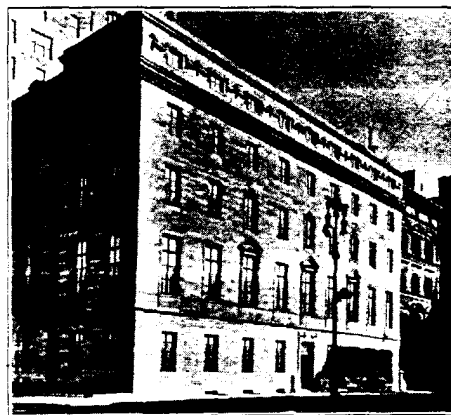
WURTS BROS. A Fifth Avenue residence, New York, which rests on lead-asbestos anti-vibration pads
