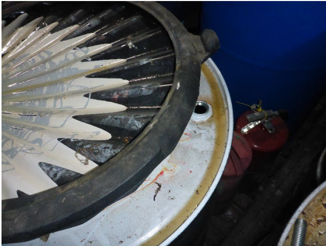
Photo 23: An open bung and hazardous waste liquid on the top of a hazardous waste storage container in the main CAA.
