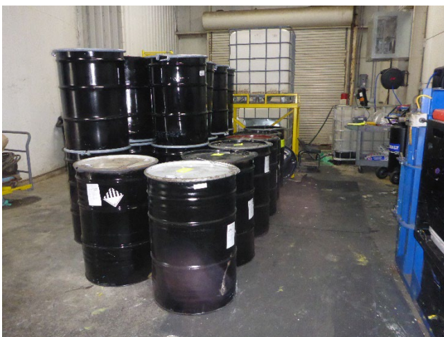
Photo 19: Six 55-gallon containers for consolidated hazardous waste debris located next to several empty 55-gallon containers, which are stacked two high, in the Fire Pump House CAA. Each hazardous waste container was closed, labeled with the words "hazardous waste", marked with an accumulation start date and identified with a two-letter customer identification code. Each container was labeled with a DOT class 9 hazard sticker, but none were marked with an indication of the hazards of its contents.
