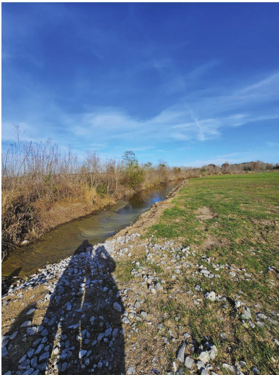
Channel for runoff from field to Contact basin
