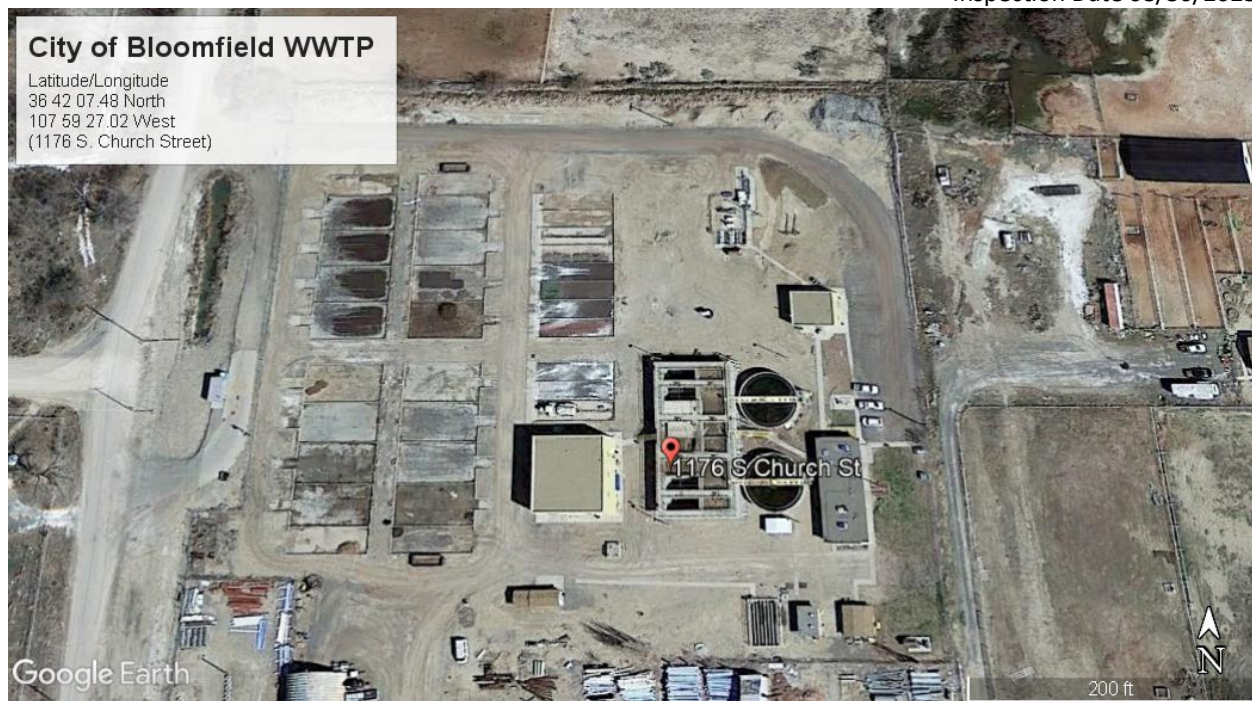
Aerial Image #1 Overall view of the existing City of Bloomfield's Wastewater Treatment Plant. Aerial from Google Earth.
