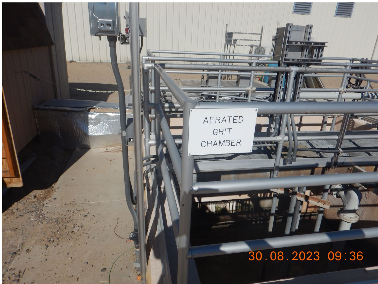
View of rehabilitated Aerated Grit Chamber. (DSCN2637). Photographed by D. Esparza
