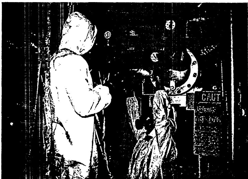
The central question remains: When is enough asbestos removed to ensure a practical and sufficient margin of safety?
