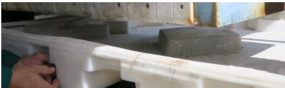
Photo 77: Inspectors observed filter cake waste accumulating on top of the “lid”, this waste was open to the environment.
