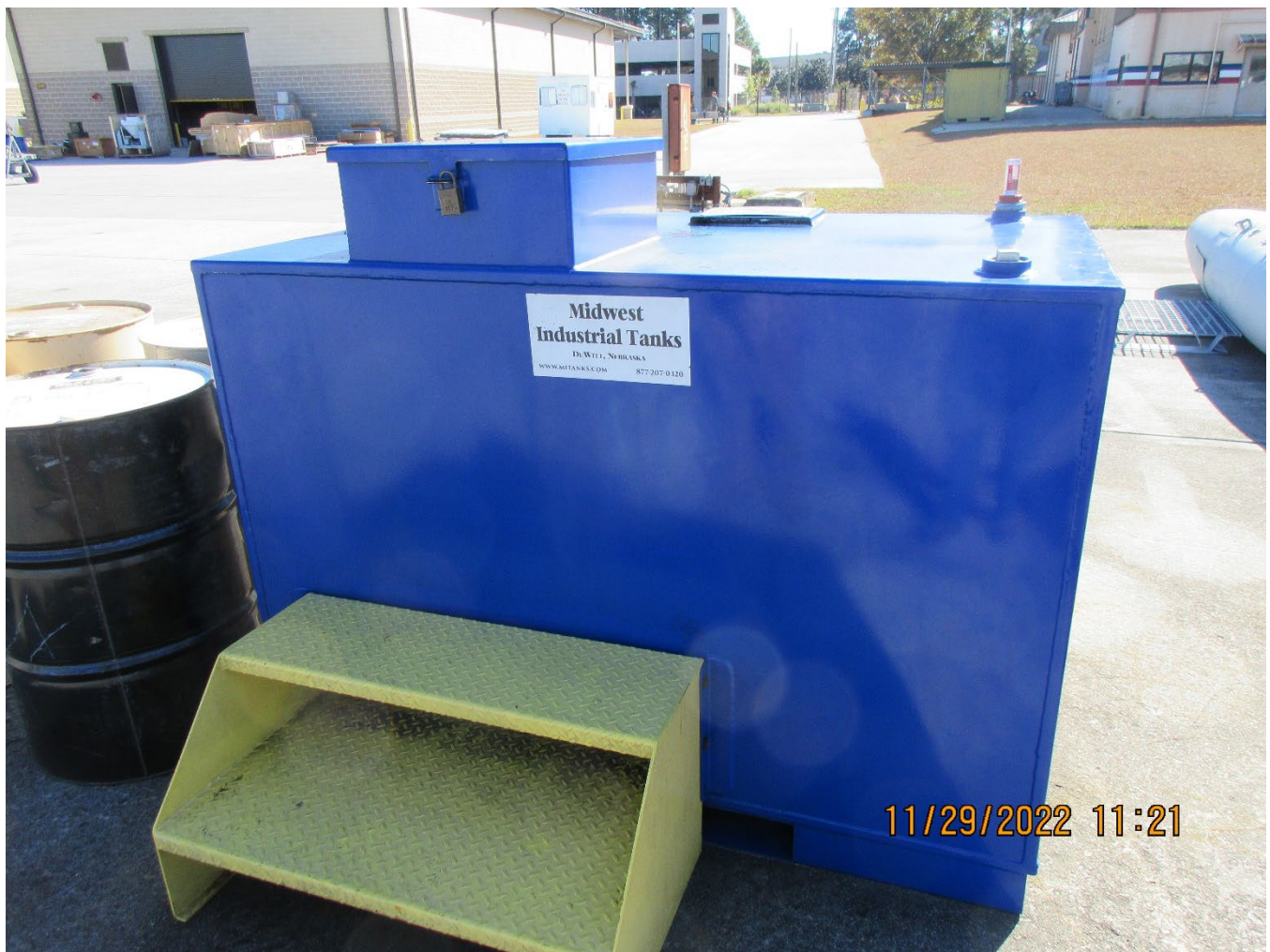
Photo 3 – Used Oil Container on flight line outside Hanger 414
