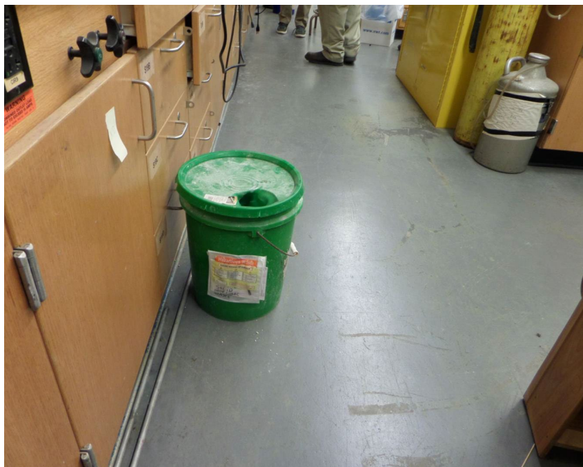
Photo-10 Chemistry Physics Building – CP34 Indication of hazards of contents not marked, Container in bad condition
