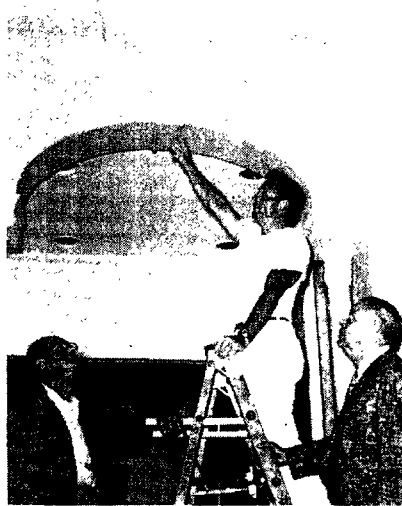
● FROM RIGHT are Arthur D. Hoppe, president of the firm; Wayne Beatty, plastering foreman; Jack Hasley, vice president and field superintendent; Wayne is showing how he joined an ornate piece of staff work to run mold—with perfect alignment
