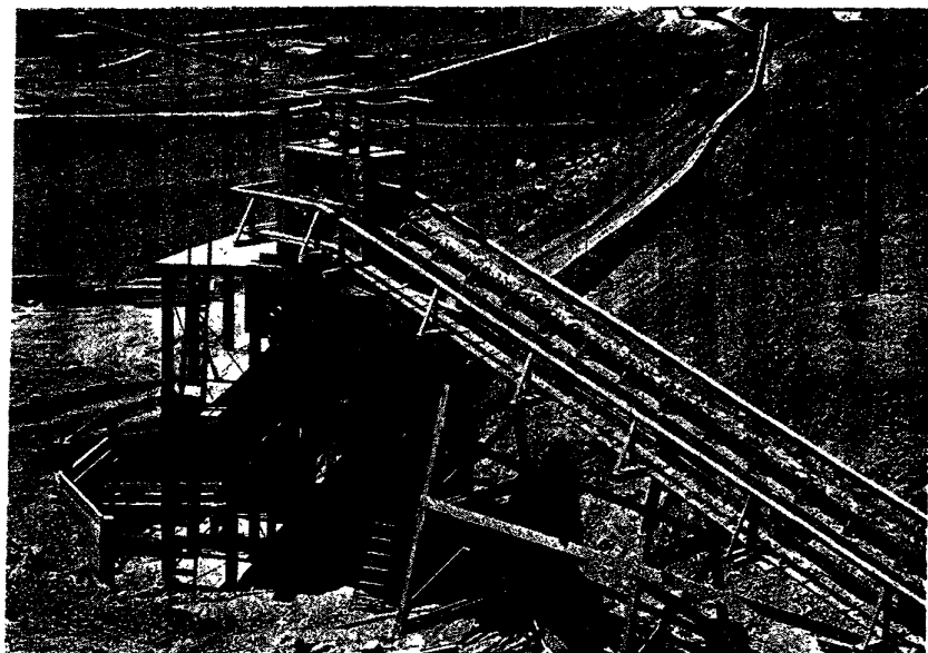
The Natividad plant of the Permanente Metals Corp., showing the main conveyor belt from the dolomite quarry. The main calcining plant (center) delivers the finished product by conveyor to the storage bins (left of center).
