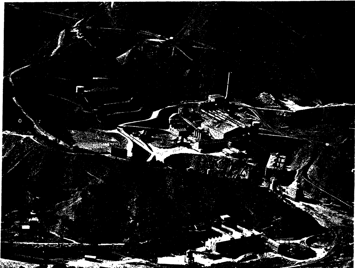
Aerial view of the Permanente Cement Co. plant near San Francisco.
