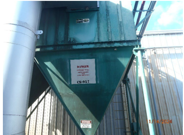
Picture 9 – Blast Media Booth CLEMCO baghouse
