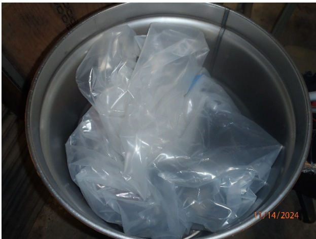
Picture 31 – Breaker Shop Special Waste – Asbestos Arc Shields
