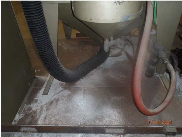
Picture 25 – Breaker Shop Zero Blast Cabinet spilled media
