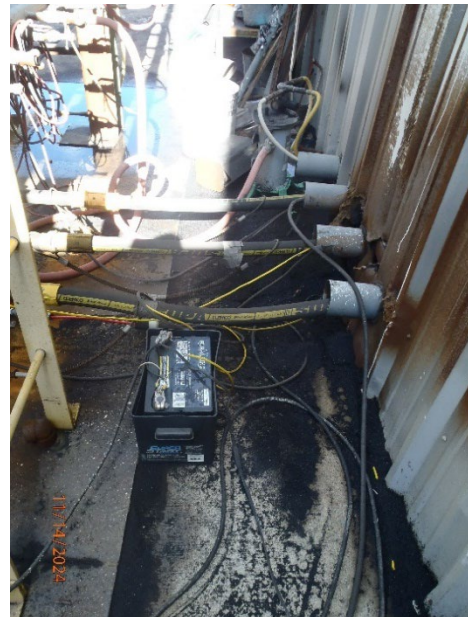
Picture 46 – Shop 2 Blaster Shop lead acid battery in water
