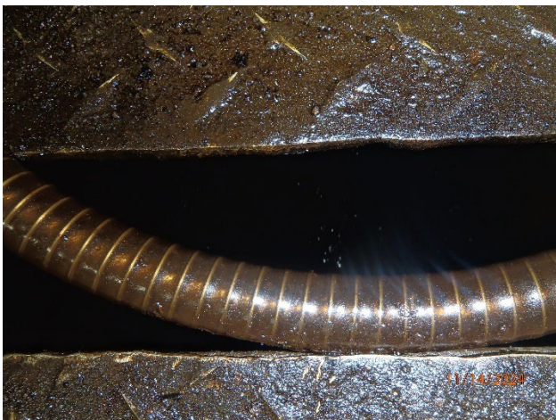
Picture 38 – Shop 2 Compressor Room condensate collection box oily water
