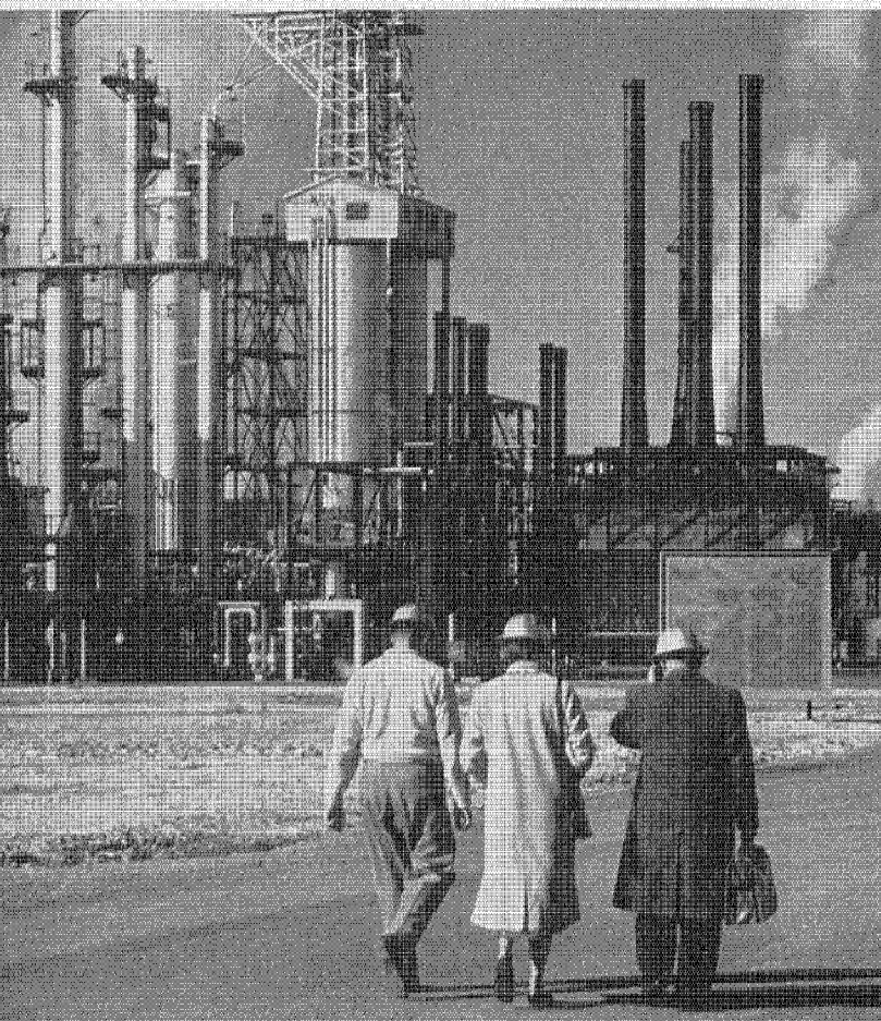
Stockpiles of black Gilsonite ore, above, are turned into high octane gasoline and petroleum coke in refinery near Grand Junction, below. A catalytic cracking unit is at the left, a delayed coker at right.
