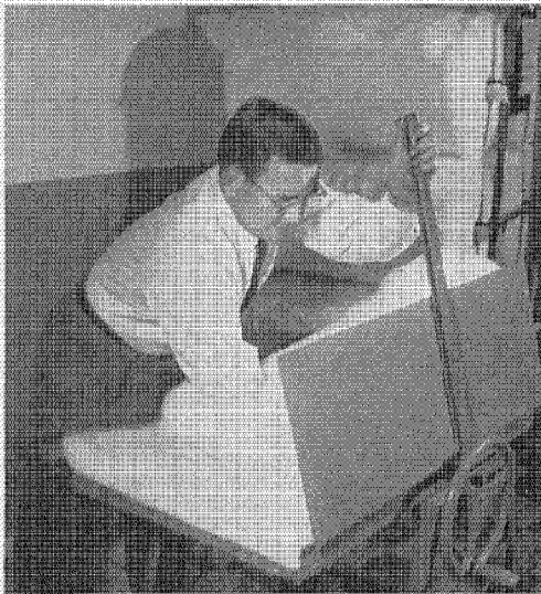
Fibers are compressed here in hand-operated machine duplicating commercial process.
