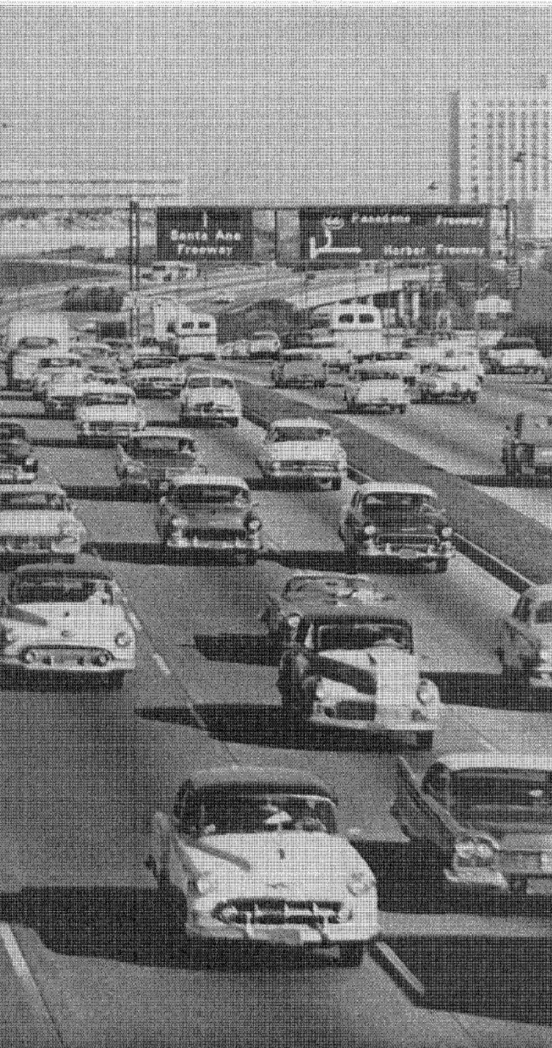
Motorists in Southern California had a beef: their tire sidewalls were cracking severely. Ozone was the culprit, neoprene the answer.
