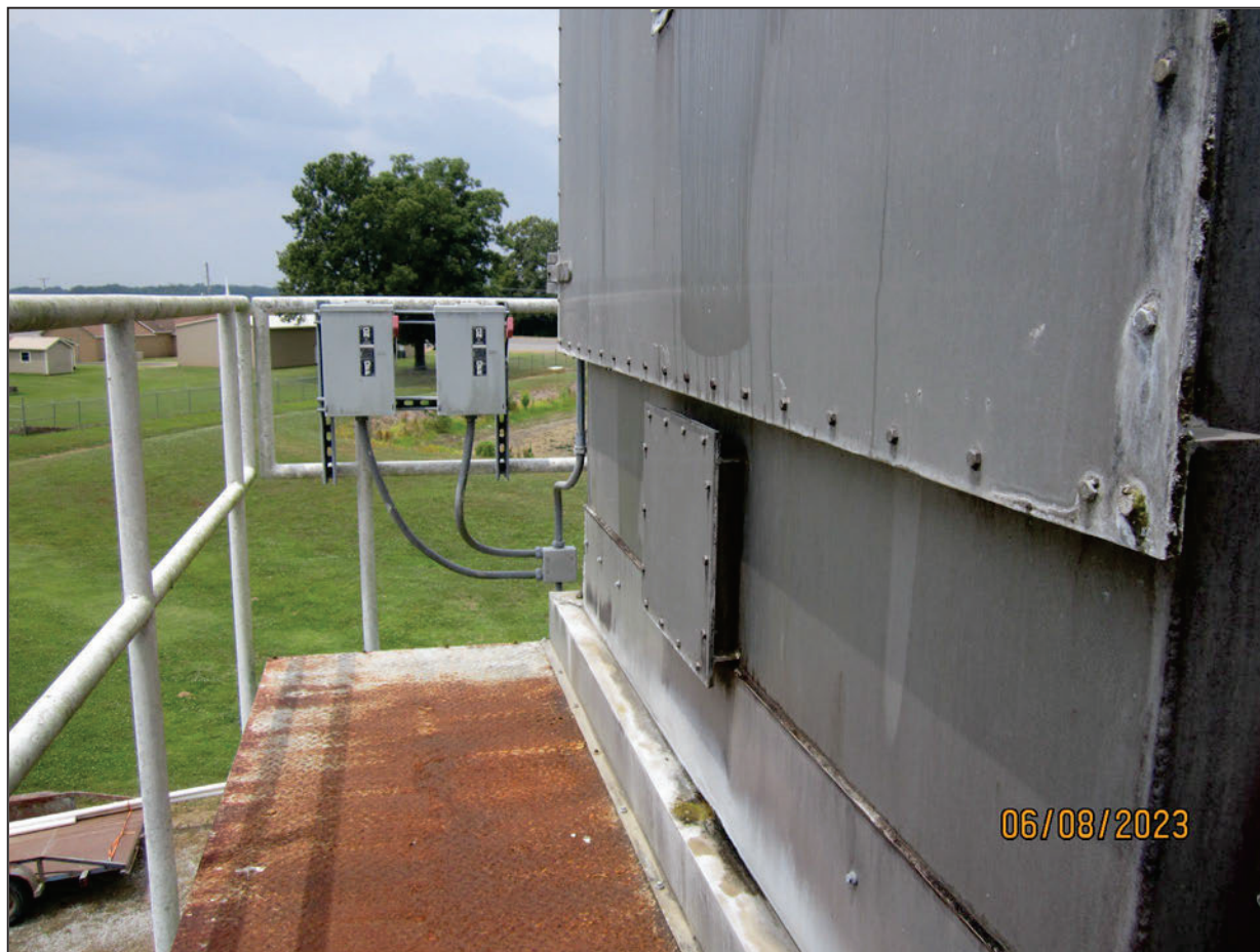
Photograph 7. Water Treatment Plant, Aerators View of one of the aerators and the control panel for both units. Both units were operating.
