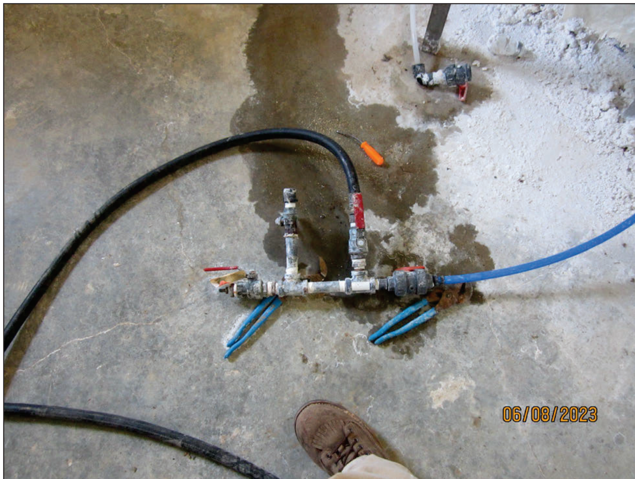
Photograph 13. Water Treatment Plant, Chemical Storage and Pump Area View of current maintenance being conducted on tubing supporting the delivery of treatment chemicals to the process areas. It appeared that the team was using PEX piping in their current modifications to the chemical delivery system. The delivery system was resting on the floor of the chemical storeroom. There was dried chemical residue in various areas of the room.
