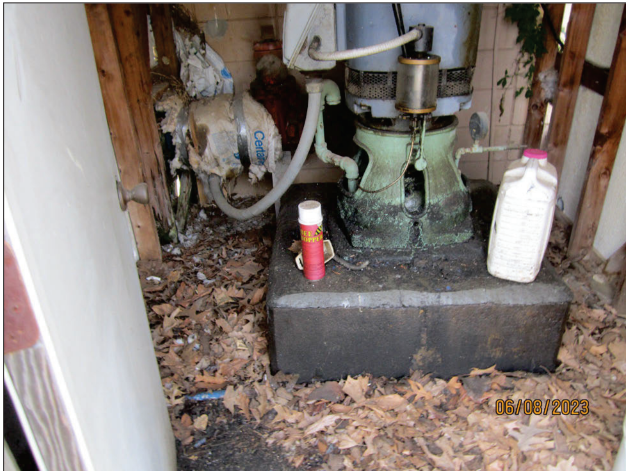
Photograph 2. Well #1 View of Well #1, that was located within a shed. Components of the raw water lines were wrapped in insulation. There was a can of bee spray and an unmarked container resting on the well pedestal. The pedestal and motor stand structure appeared to have a layer of oil. There was an accumulation of leaves and some debris surrounding the well pedestal.
