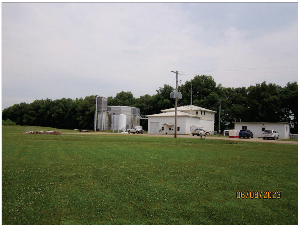
Photograph 6. Water Treatment Plant View of the aeration and clarifier structures, the chemical and filter building and the valve building supporting the clearwell's operations.
