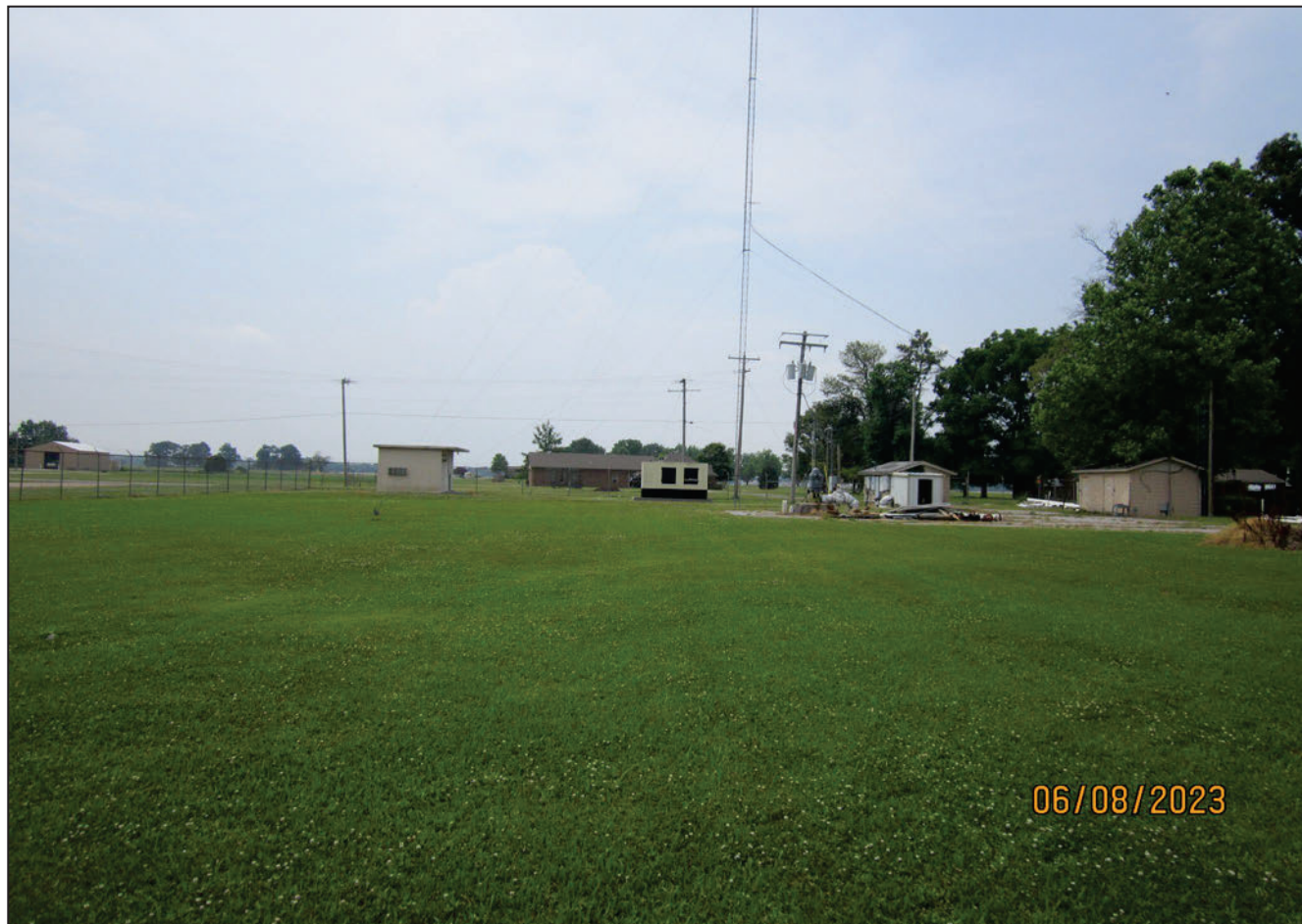
Photograph 1. Fitzgerald Crossing Well Field View of the Fitzgerald Crossing well field and backup generator. The well field was surrounded by a locked perimeter fence. There was a private residence located on the fence within less than 100 feet of all wells.
