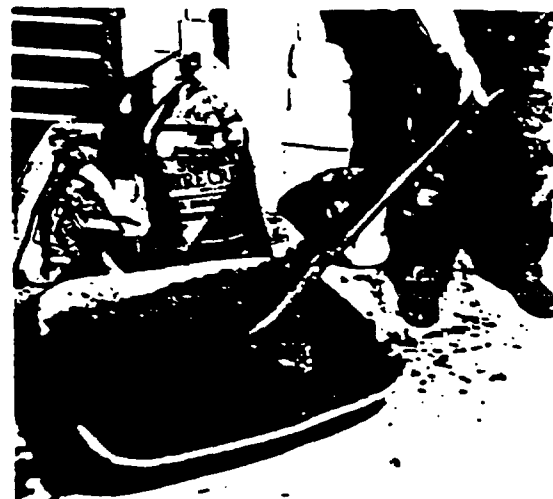
Firecrete is handled as easily as ordinary concrete. Be careful to use the right amount of water.
