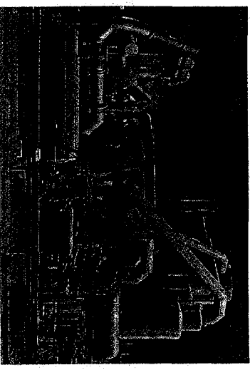
New sulfuric acid plant, shown in model, is almost completed at the Warners plant in Linden, New Jersey. A sulfur recovery unit also is being built at Warners. Both will significantly improve air quality by substantially eliminating sulfur dioxide emission.
