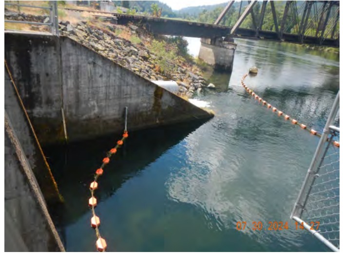
Photo #:02 (DSCN3824) Description: Facing west, photo of intake water location from North Fork Clearwater River.
