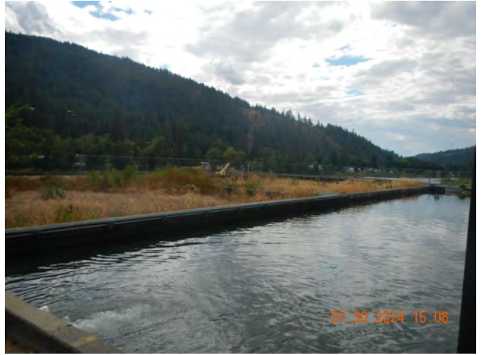
Photo #:10 (DSCN3832) Description: Facing southwest, photo of the OLSB and adjacent drying beds.
