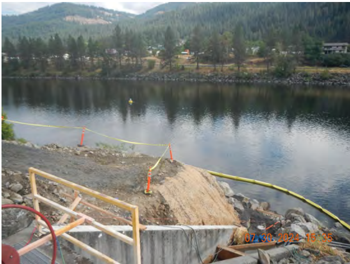
Photo #:15 (DSCN3837) Description: Facing south, photo of the construction area for the Steelhead release pipe (Outfall 004).
