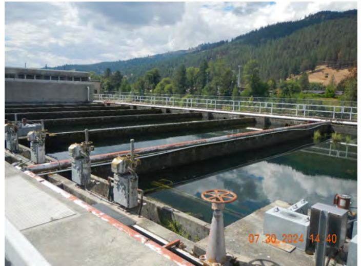
Photo #:04 (DSCN3826) Description: Facing north, photo of the System I and nursery clarifiers.
