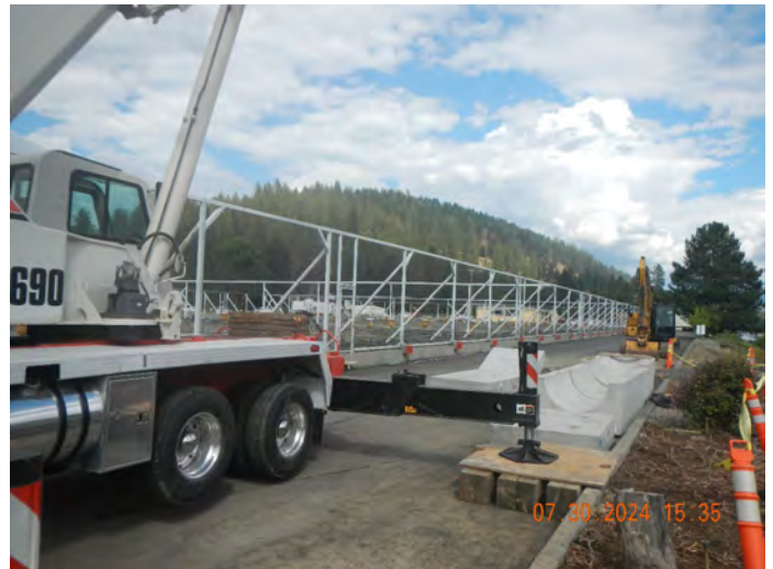
Photo #:16 (DSCN3838) Description: Facing east, photo of sections of the new Steelhead release pipe (Outfall 004).
