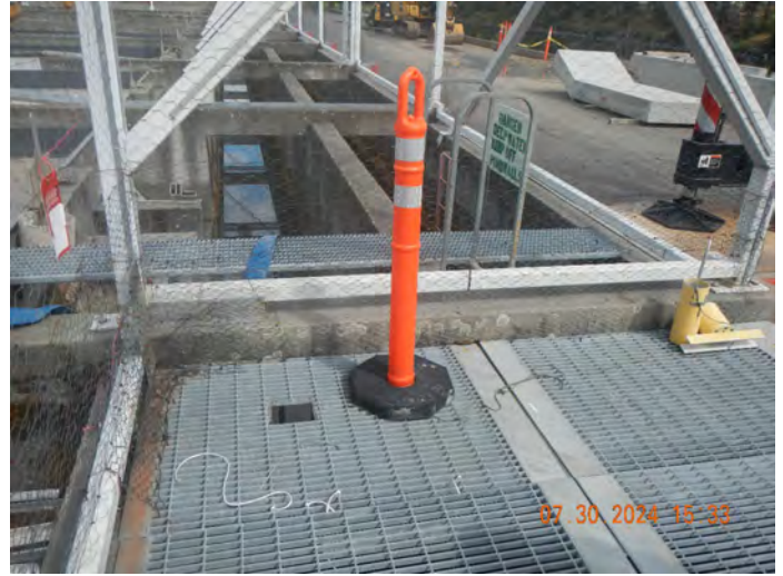
Photo #:14 (DSCN3836) Description: Facing east, photo of sample location for Outfall 004 to the mainstem Clearwater River.
