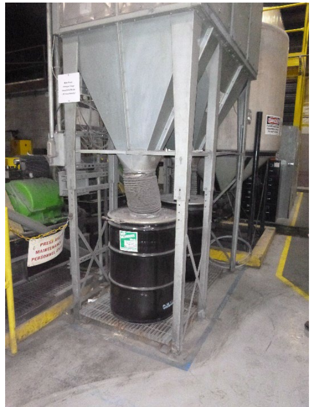
Photograph 32: Filter Press Sludge.
