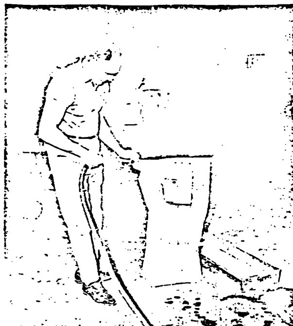
FIGURE 3. A proposed method to eliminate a major source of dust at construction sites has been the development of a plastic mixing bag for asbestos cement. Bags are partly filled with dry cement at the factory. Water is added on the job through a valve at the top of the bag which accommodates the nozzle of a hose, and the result is mixed up in the bag.
