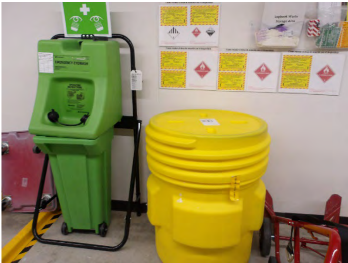
Photograph Two (2): Eye washing station and spill kit
