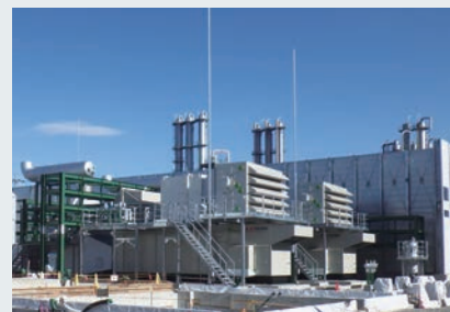
Gunma Complex (Gunma Prefecture), which is increasing its electricity self-sufficiency by adding gas turbines for power generation
