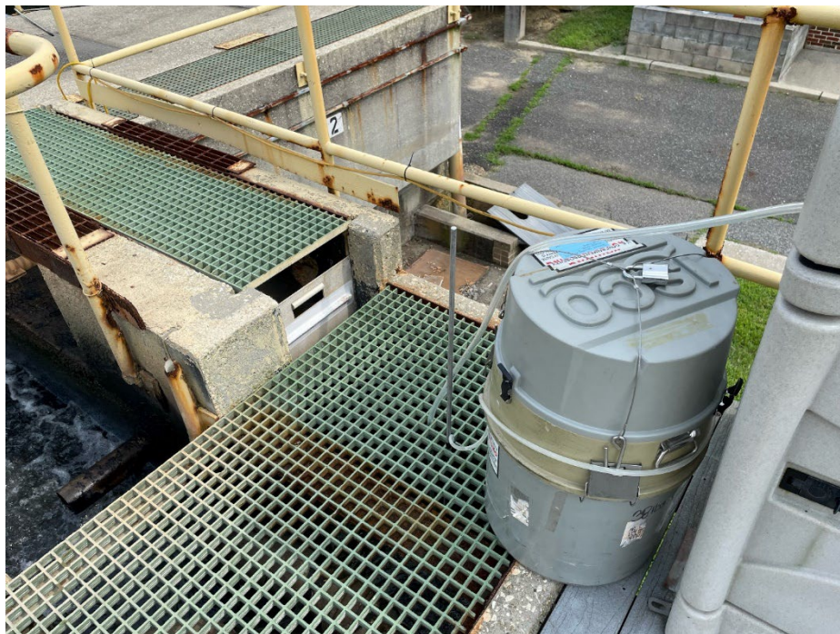
Photograph 3: EPA automatic composite sampler was setup at the influent monitoring location.
