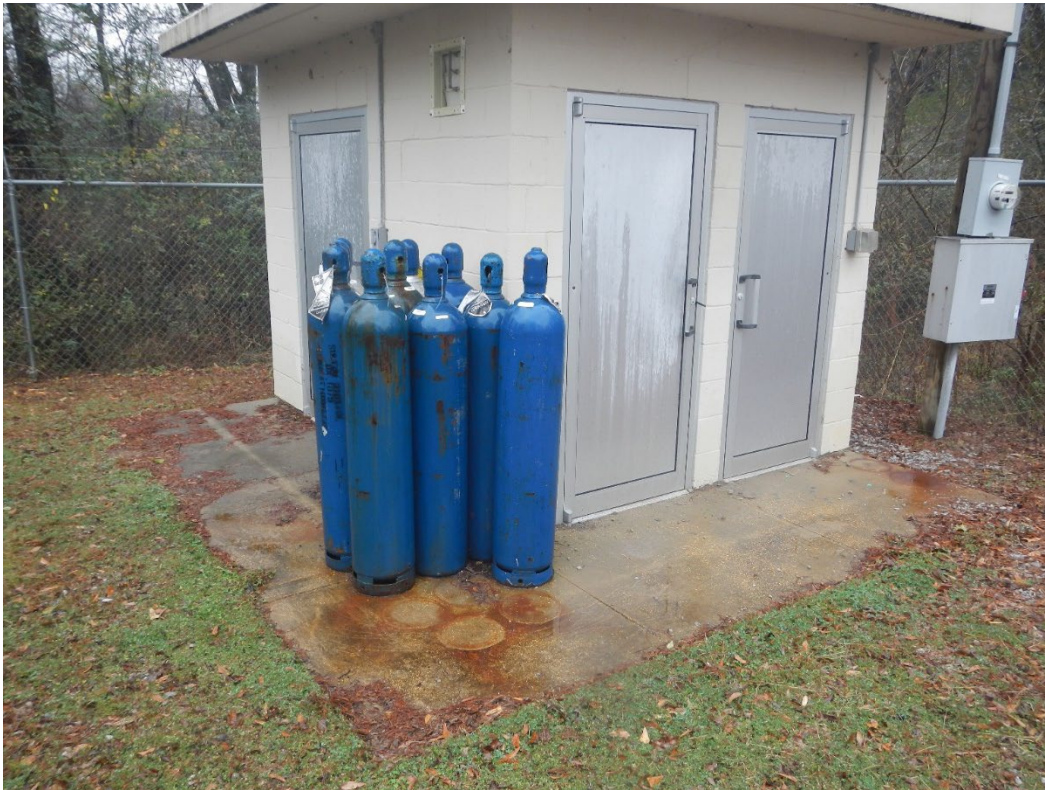
Figure 13: Empty and partially empty chlorine tanks
