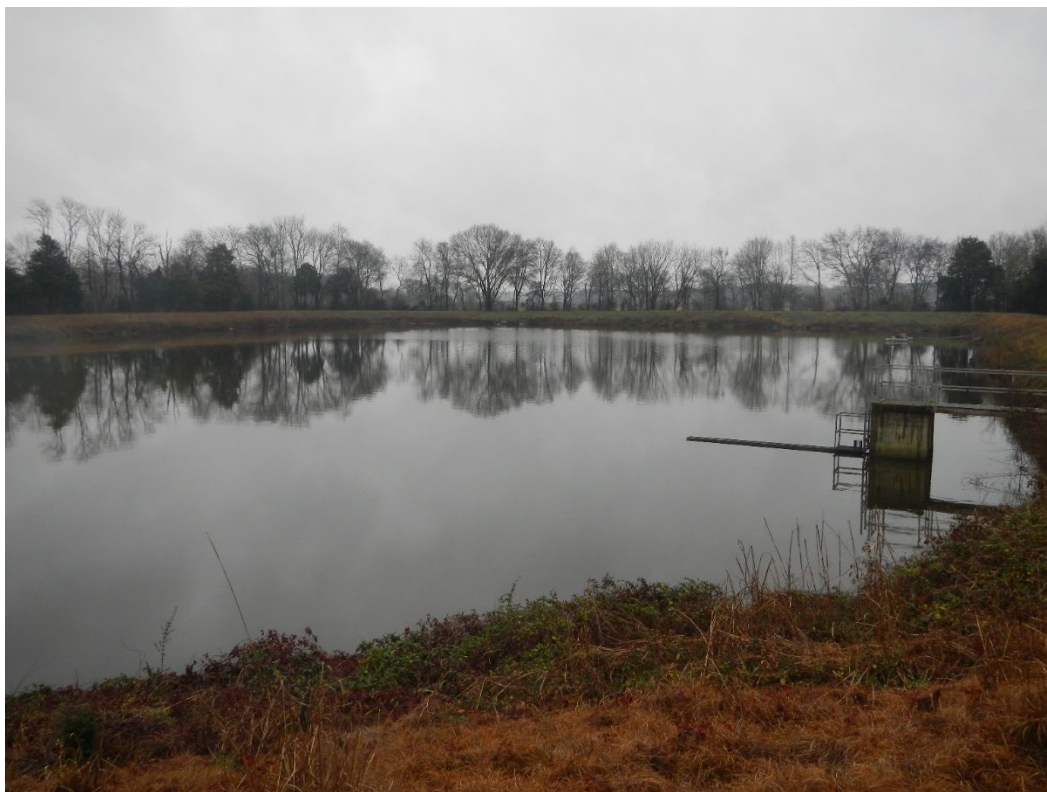
Figure 7: Shannon POTW West lagoon with effluent structure.
