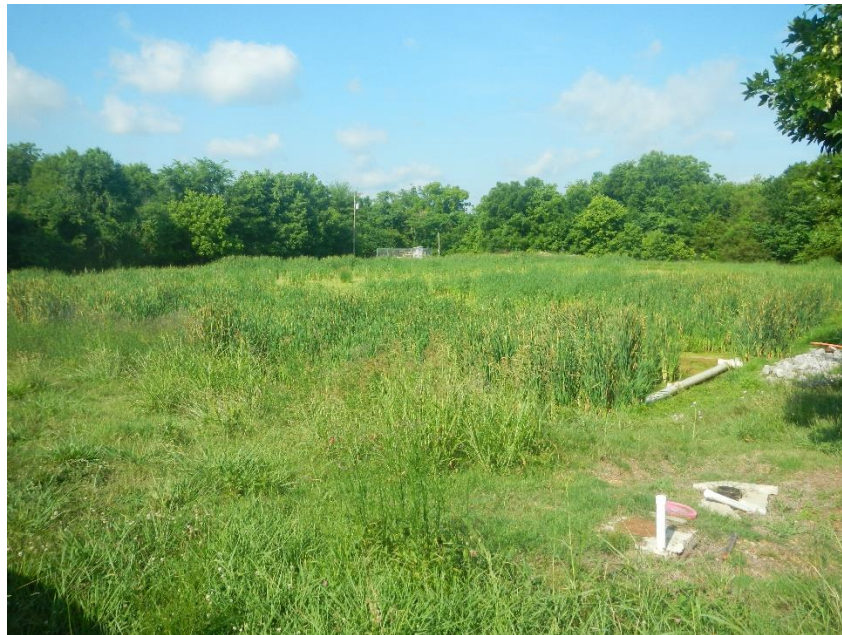
Photo 4. Constructed subsurface flow wetland growing bull rush. Chlorination structure visible in background.
