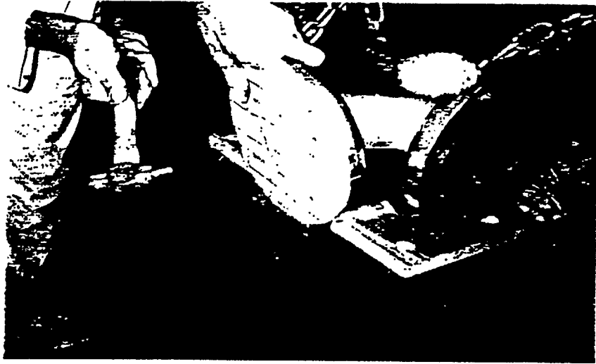
-Photo 3- Shaping of gasket material at center portion. Fitting #10D is shown.
