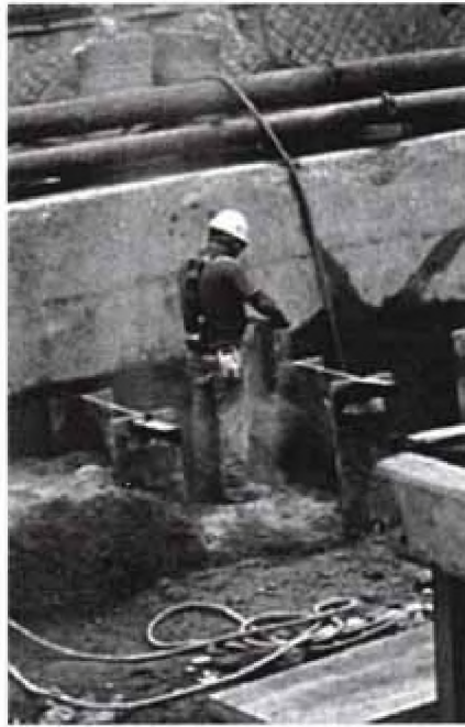
Figure 2. Construction worker on Big Dig wears air sampling monitor to test for silica exposure.
