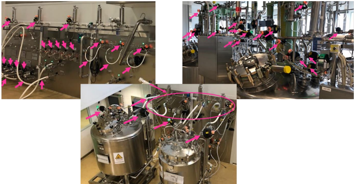
Figure 3 Formulation area, pink arrows mark membrane valves.
