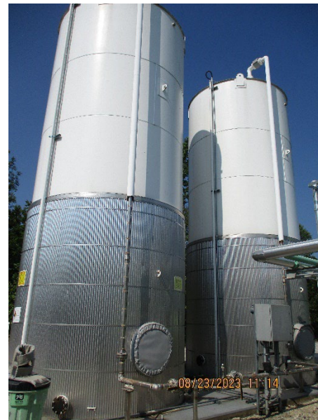
Photo 4: T-1 and T-2 hazardous waste tanks. 15,000-gallon double-walled ASTs.
