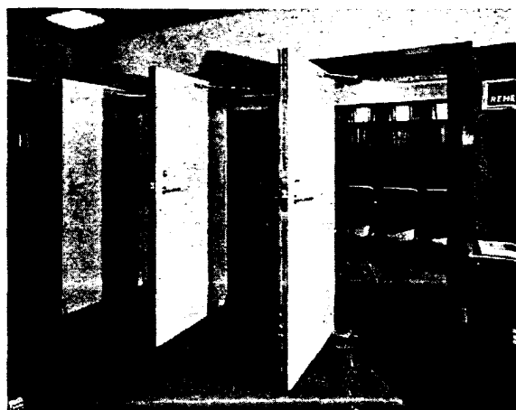
Lead-lined sound-proof doors, N.B.C. Studios, Radio City.
