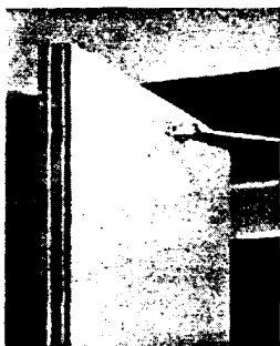
Detail of sound-proof door with edges of lead sheets visible.
