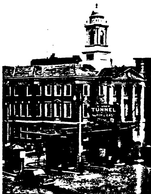
BOSTON'S SUMNER TUNNEL is a $19½ million mile long under-harbor short cut North and East. Over 11 million vehicles used it last year, with summer traffic especially heavy.
