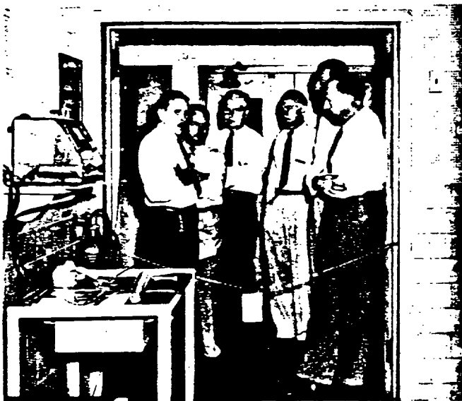
Observing a single-cylinder engine equipped with radioactive piston rings for investigation of wear are D. J. Winter, British American Oil vice president; C. H. Tew, Canadian Oil Companies; O. B. Lewis, Ethyl Corporation of Canada Limited vice president; C. E. Carson, Imperial Oil director; and D. W. Simmons, also of Imperial. Benjamin Brewster (left) explains tests.
