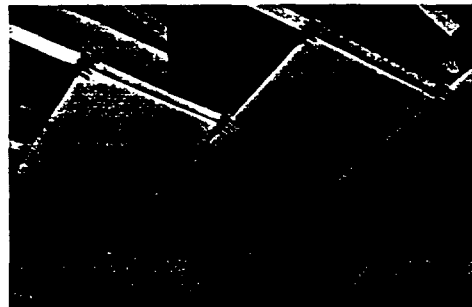
The best practice in applying Rocklath calls for Cornerize on all interior corners, corner bead on all exterior corners. Striplath reinforcement at windows, mantels, and doors; also at end joints of Rocklath on ceilings and lengthwise of the room at the center of ceiling.
