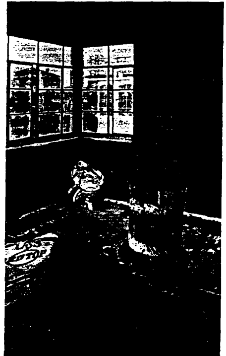
Ventilation and heat are properly provided. There is no fog on the windows. The salamander is throwing off enough heat to maintain the necessary drying conditions. It is placed in the center of the room, so that the plaster will not be exposed to excessive heat. If it is necessary to place a salamander near the wall, Insulating Rocklath should be placed between, with the foil side toward the salamander. This will protect the plaster.
