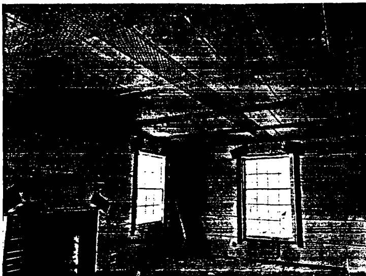
The best practice in applying Rocklath calls for Cornerize on all interior corners, corner bead on all exterior corners. Striplath reinforcement at windows, mantels, and doors; also at end joints of Rocklath on ceilings and lengthwise of the room at the center of ceiling.
