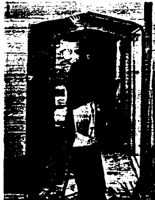
It goes up quickly! One continuous piece of Red Top No. 4-A Flexible Corner Bead was used to form the right side of the arch. Left half of arch is ready for nailing and splicing to right side of arch.
