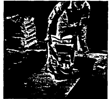
Empty contents of lime bag by placing the open end in the water on the bottom of the box as in photograph at left. Withdraw bag immediately as shown at right.
