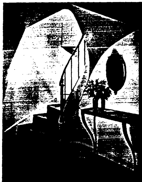
Metal lath and plaster are vital to obtain notable decorative effects such as this. USG Jr. Diamond mesh is readily shaped to reproduce any architectural design. After the job is completed, it provides reinforcement that gives maximum protection against cracking. Plasterers who encourage architects to include details of this type in their work are strengthening their business foundation. The Strong residence, William Alderman architect.
