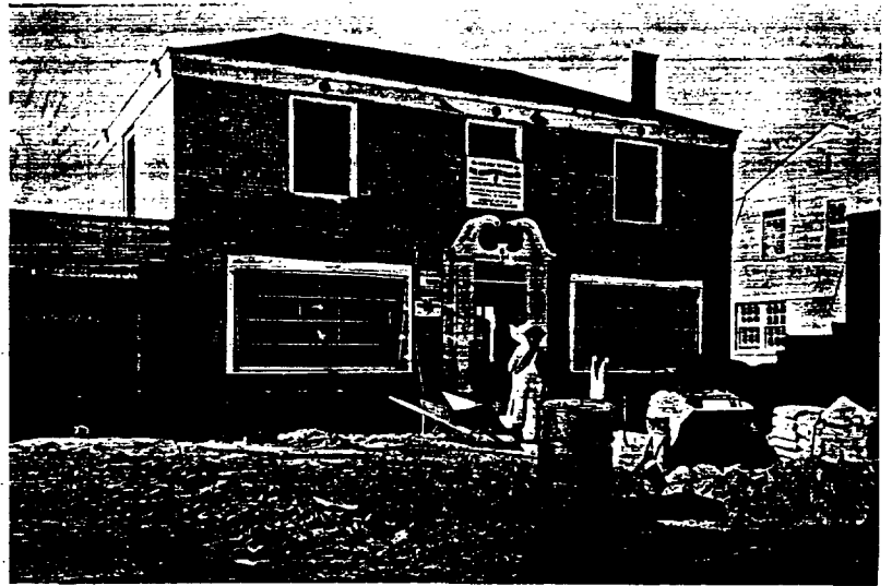
This is an ideal set-up for efficient work. The mixer or mixing box is directly in front of the door to the house and it is only a few steps from the plaster box to the entrance. Red
