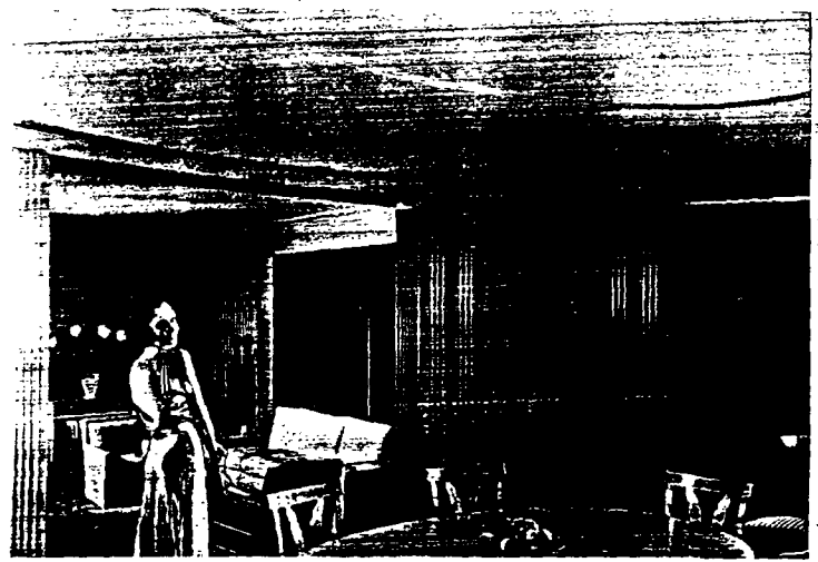
This notable example of a modern interior vividly illustrates why plaster is still the long favorite as an interior finish. Obviously, metal lath is essential as a plaster base for work of this character and its flexibility, together with the reinforcement which it provides to the wall, assures the owner an interior that will have long life. The added cost for the decoration, which includes a formed, suspended ceiling and curved walls with ornamental work, is estimated at about $75. Far more might have been spent for wood paneling or other special decorations that would have been much less effective. McStay-Jackson, architect.
