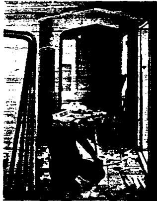
This arch or any other can be "beaded" quickly with Red Top No. 4-A Flexible Corner Bead. The Bead is formed to curvature desired by snipping one side of flange—only \frac{3}{8} " of metal—and bending to fit.
