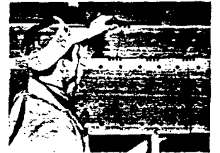
Ends of Rocklath must break between joints on ceiling as well as walls. As application proceeds, a W-22 clip is placed at each joint.
