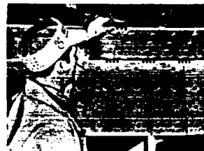
Ends of Rocklath must break between joints on ceiling as well as walls. As application proceeds, a W-22 clip is placed at each joint.
