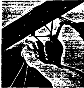
After runner track is in place, studs are tied to ceiling track with attachment shoes, which permit upward adjustment of 4 inches over actual stud length.
