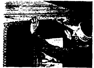
A splice joint is made by inserting a nail with the head cut off between the two sections of Corner Bead. Edges are then crimped together, thus "welding" the two sections into one secure unit. An 8 penny finishing nail is just right for this purpose.
