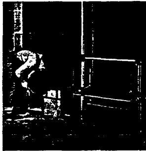
It is not necessary to have a snug fit of the runner track where pipes and ducts pass through. Track is flexible — follows contours of irregular surfaces.
