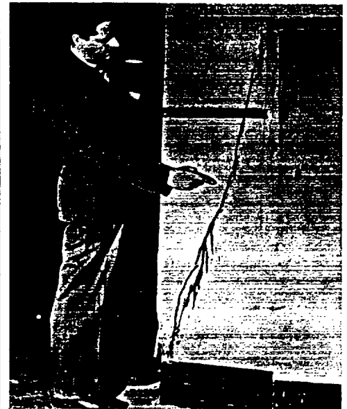
So the plaster cracks! Plasterers know that no plaster base will correct structural faults. In the illustration above, the crack is apparently due to structural movement. In most cases it is possible to point out to an owner where the trouble lies—what actually caused the crack. By explaining to owners who complain of plaster cracks that no interior wall finish will eliminate this trouble, plasterers will increase public appreciation of good plastering.
