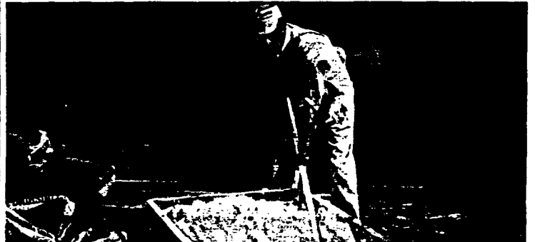
To allow lime to get completely wet, wait 15 minutes after last bag is emptied. Then hoe the lime to the desired consistency, add gauging plaster and use. Screening of putty through \frac{3}{16} " to \frac{1}{4} " mesh screen is recommended for best results.
