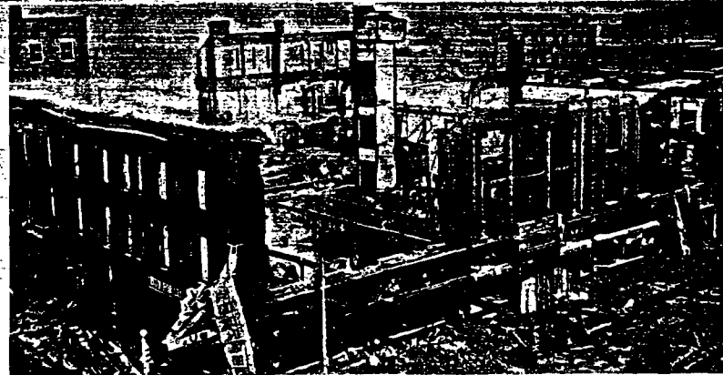
(Billings Gazette Photo) The result of the worst fire in the history of Billings, Montana. Notice that in spite of the terrific heat and smoke, the plaster showed little discoloration.
