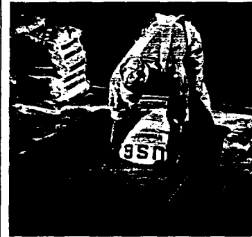
Empty contents of lime bag by placing the open end in the water on the bottom of the box as in photograph at left. Withdraw bag immediately as shown at right.
