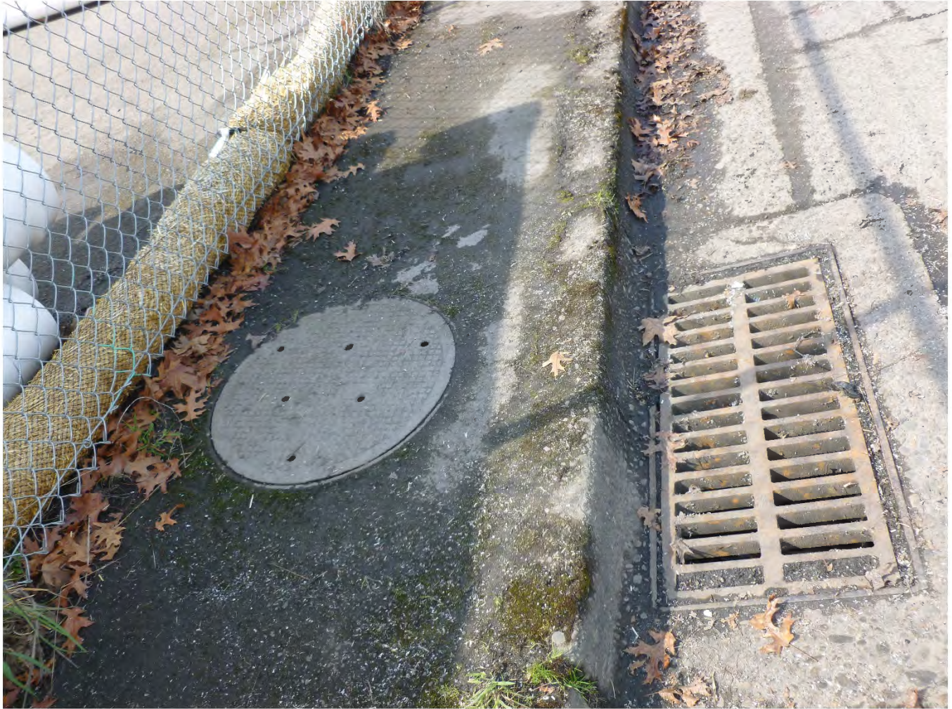
Photo 5 / P1000796 – Storm Drain, east side
