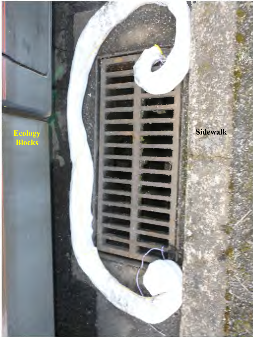
Photo 9 / P1000799 – Storm Drain, west side
