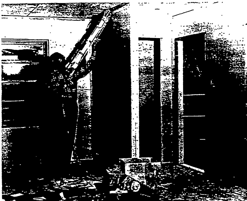
Hormuth's father, Marion, uses old-style drywall taping tool which operated on battery power. Picture was taken sometime in mid-1940's, according to Hormuth.
