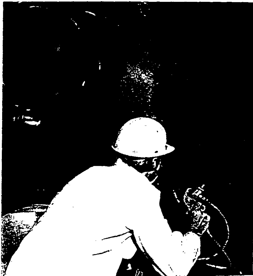
Glass is sprayed on the outside of the vessel, too, before its first firing.
