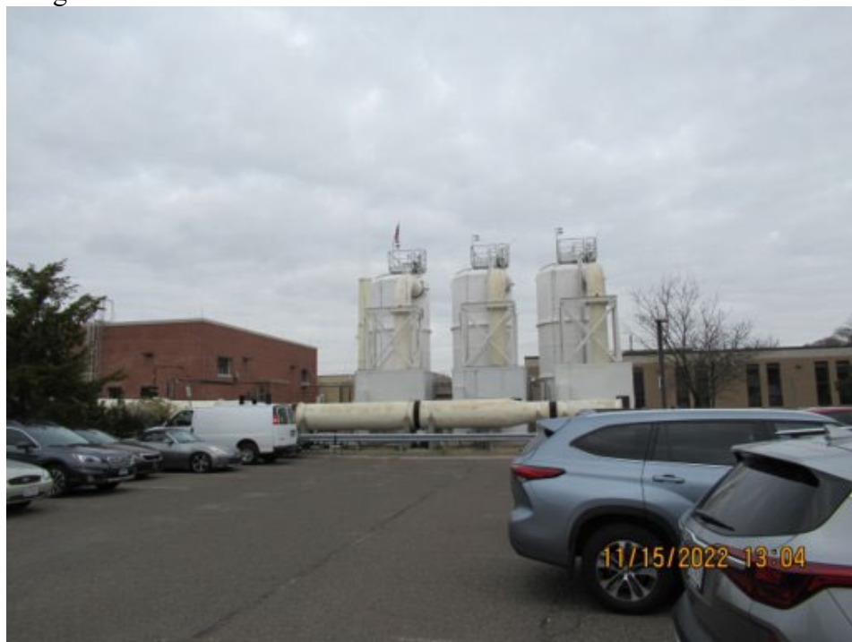
Photograph #1 – Primary tank odor control building in foreground, administrative building in background
