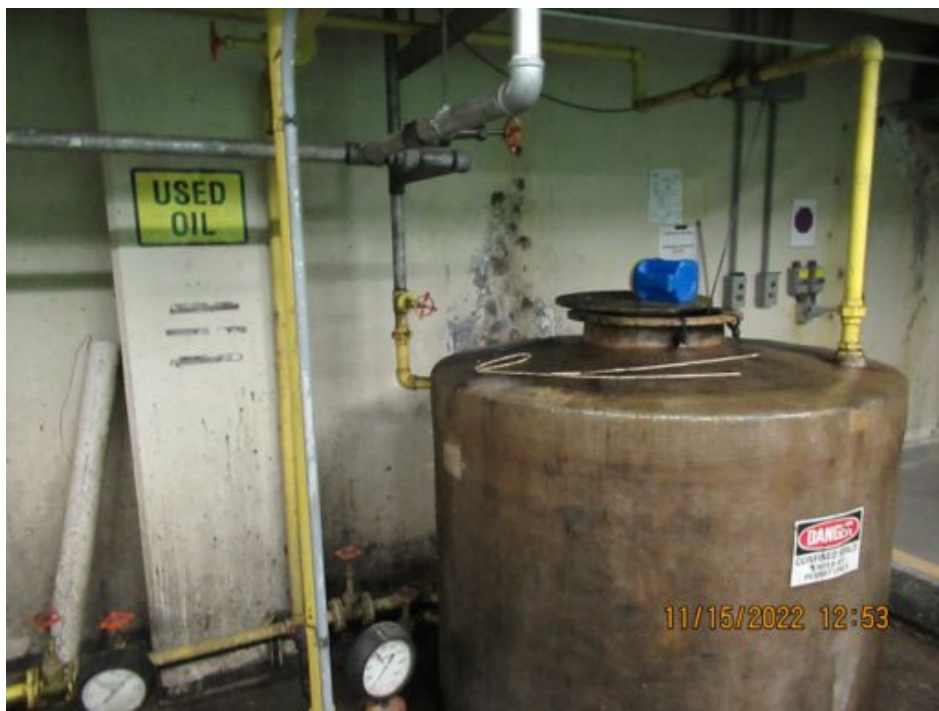
Photograph #6 – Used oil tank
