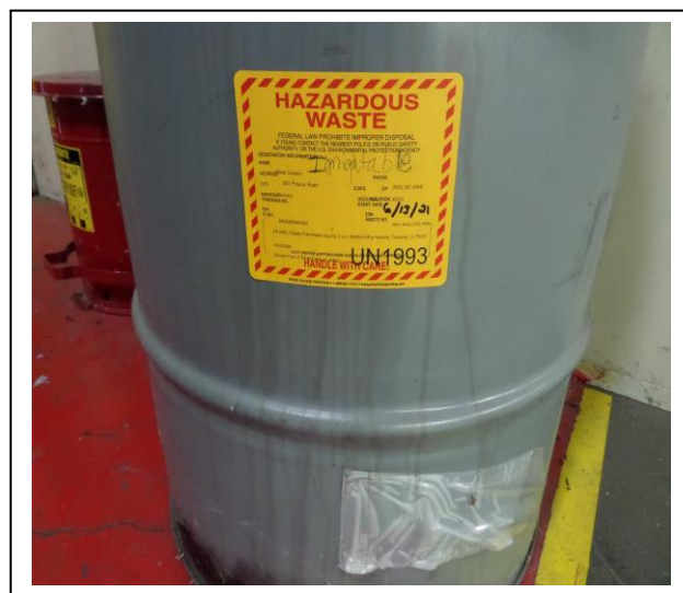
Metal Coaters. Core Room/Laboratory. The container was not marked or labeled with a hazard indicator. Photograph 2 taken at 10:58 a.m.
