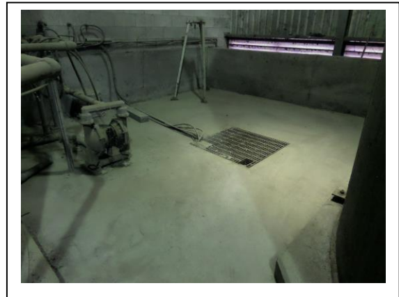
Metal Coaters. Solvent Storage Room. Inspectors observed floor level concrete sump. Photograph 20 taken at 12:08 p.m.
