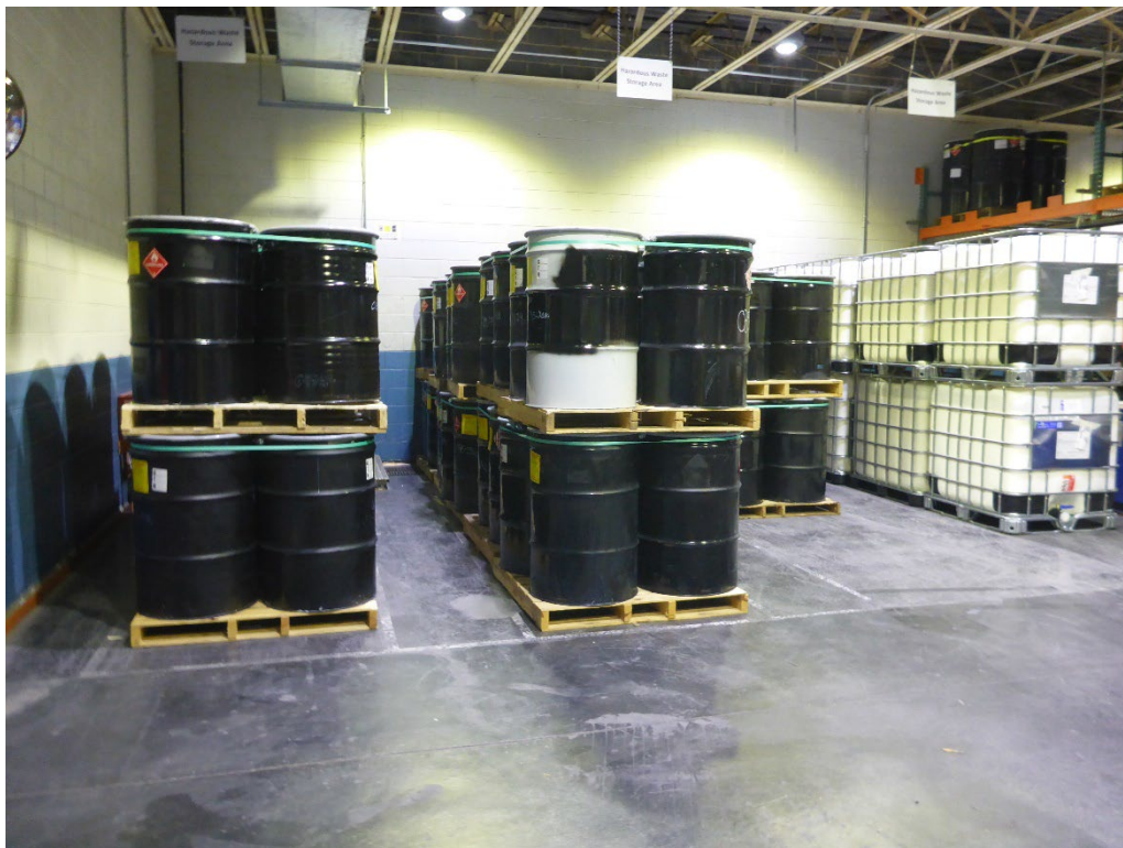
Photo 19: CAA located in Drum Storage Area 2. The floor has been painted to define individual rows for storing pallets of hazardous waste containers. The inspectors observed approximately one-hundred 55-gallon drums of hazardous waste arranged in three rows of wooden pallets.
