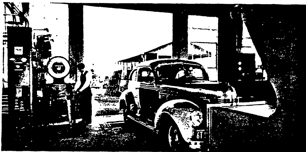
This car is bucking a gale of 85 miles an hour — blown through the large duct facing it.
