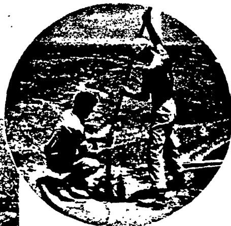
In shallow holes, the shot is lowered by means of poles which hook together. When the charge reaches bottom, a simple twist unhooks the lowest joint and the poles are recovered.
