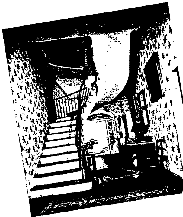
Front door and unusual stairway at COTTAGE GARDENS, home of the Foster family. Built in the 1790's and at one time owned by Don Jose Vidal, acting Governor of the Natchez Territory at the time of Spanish evacuation (1798).
