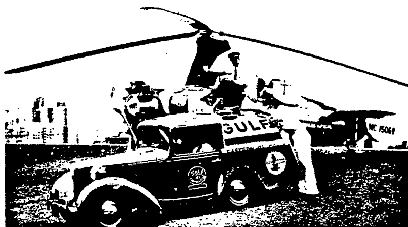
A specially constructed miniature gasoline tender fuels the Autogiro on the roof of Philadelphia's Post Office.
