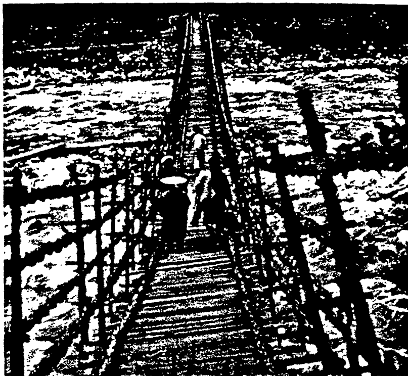
Mrs. Harkness crossed many of these swaying suspension bridges. Made entirely of bamboo, there is not a nail or rivet in them yet their bamboo cables are similar to cables of steel.
