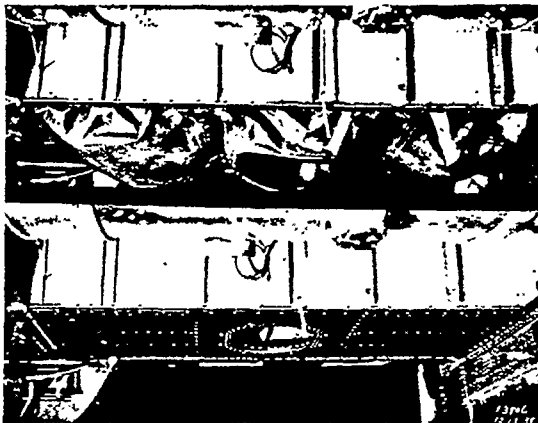
Three-cell, 185 gal. Mareng Fuel Tank in wing compartment. Above: before bottom plate is fastened in place. Below: bottom plate in place, showing hand-hole through which cells may be removed for repairs and reinstalled.
