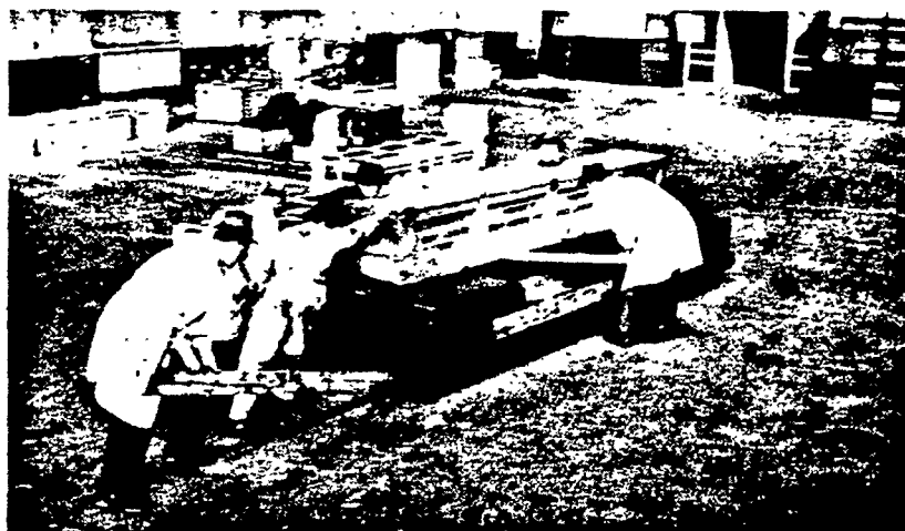
13 The all-important three-ton dynamometer is moved to its carefully selected location and acts as a foundation for the stage.
