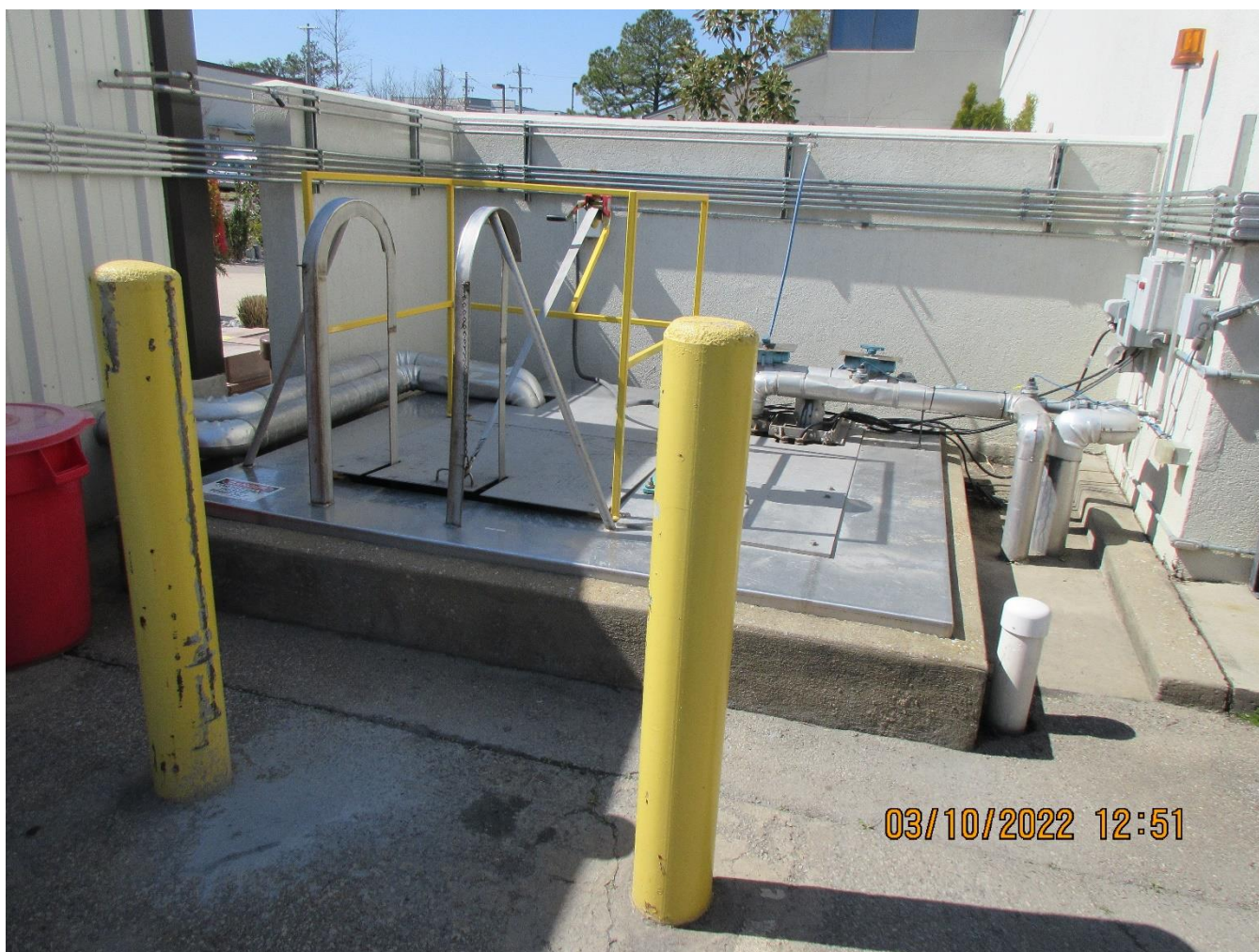
Photo 7 - Wastewater sump prior to discharge to POTW
