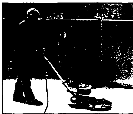
Stripping and polishing asbestos containing floor tile can cause fiber release. The EPA has prepared a new guidance document outlining safe handling procedures.
