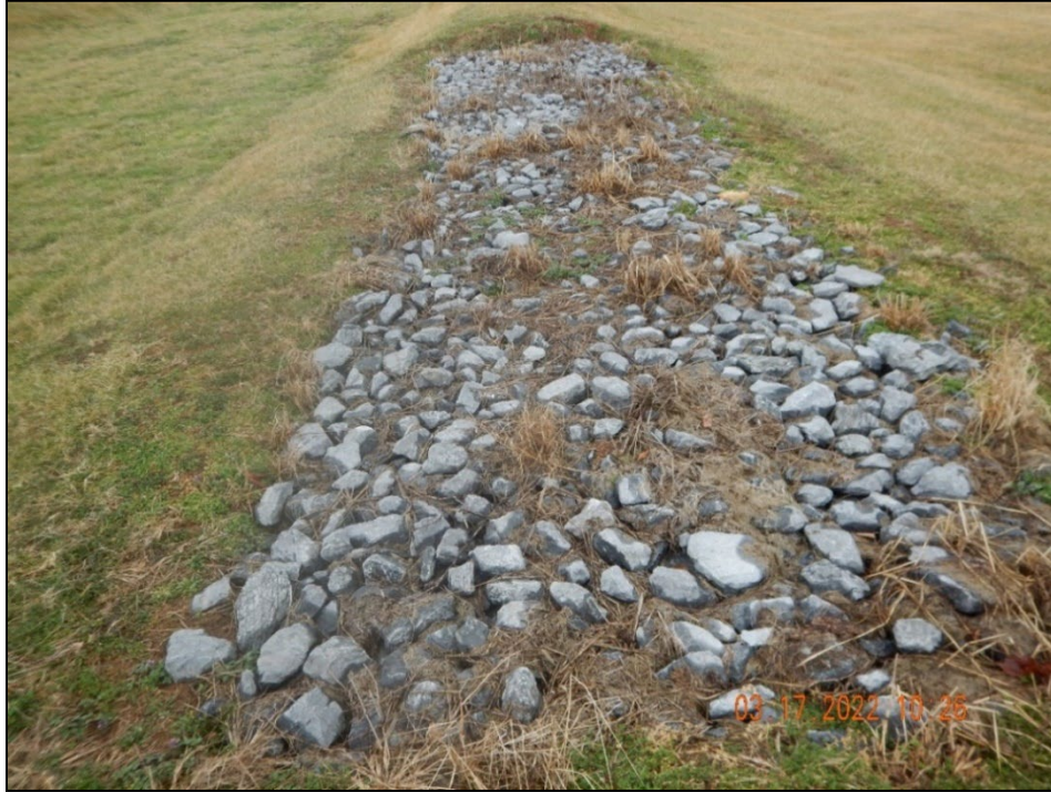
Photograph 27. Vehicle Facility Yard: (DSCN3680.JPG) View of the overflow spillway from stormwater basin 2 into stormwater basin 3.
