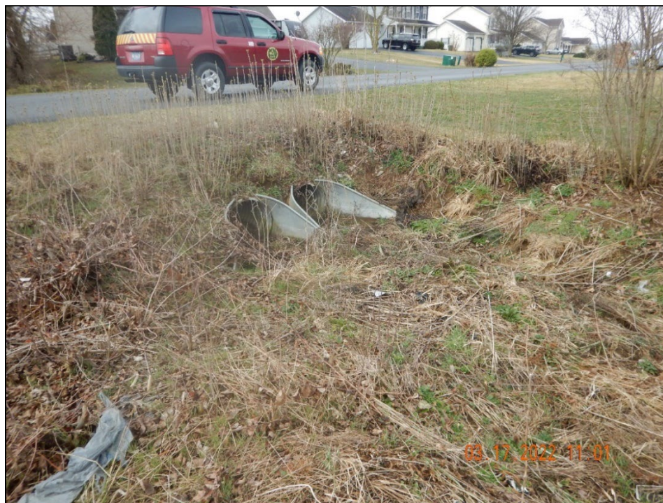
Photograph 32. Outfalls #0240 & #0245 Jason Drive: (DSCN3700.JPG) View, facing south, of Outfall #0245. No discharge was observed at the time of the inspection.
