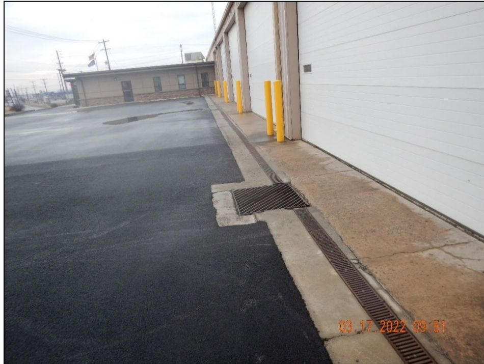
Photograph 17. Township Municipal Building: (DSCN3661.JPG) View, facing south, of drains outside of the vehicle storage garages in the Municipal Building. The drains convey stormwater to the oil/water separator and then to the sanitary sewer.
