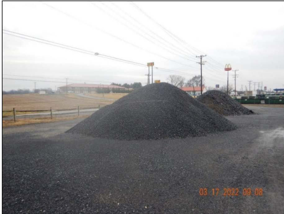
Photograph 3. Township Municipal Building: (DSCN3639.JPG) View, facing south, of aggregate material stored in the southern area of the Municipal Building. The aggregate material did not have containment measures or covers at the time of the inspection.
