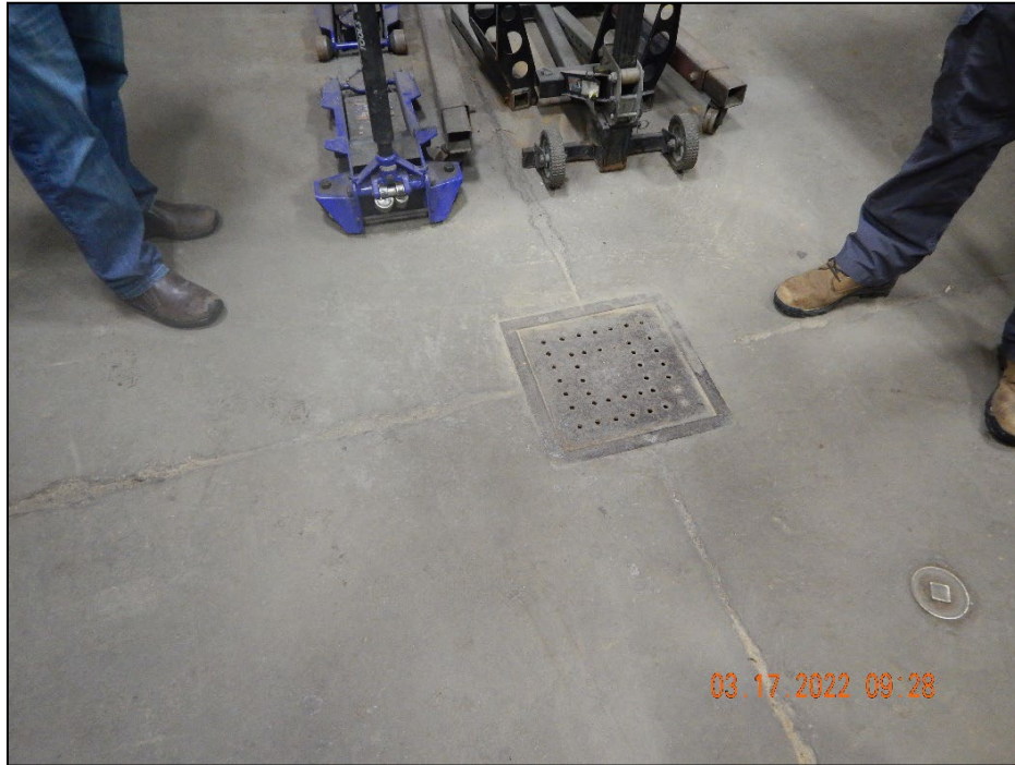
Photograph 11. Township Municipal Building: (DSCN3650.JPG) View of a drain in the vehicle maintenance garage in the Municipal Building. The drain leads to the sanitary sewer system.
