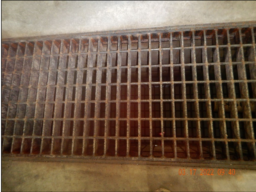
Photograph 15. Township Municipal Building: (DSCN3657.JPG) Closer view of the drain in the vehicle wash garage in the Municipal Building, as shown in Photograph 14.
