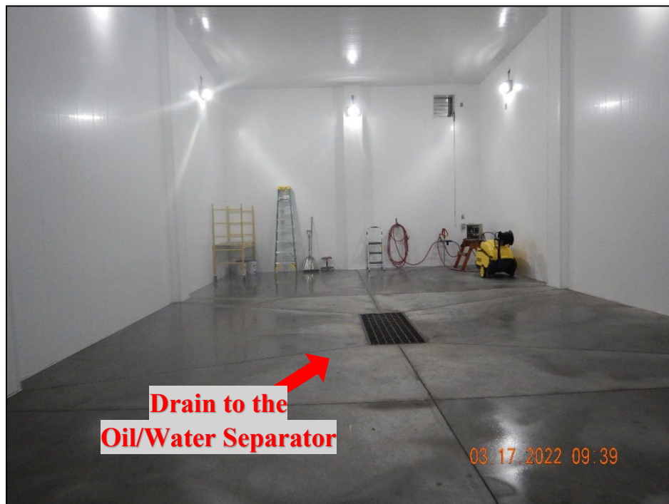
Photograph 14. Township Municipal Building: (DSCN3655.JPG) View inside the vehicle wash garage in the Municipal Building. Note the drain that leads to the oil/water separator.
