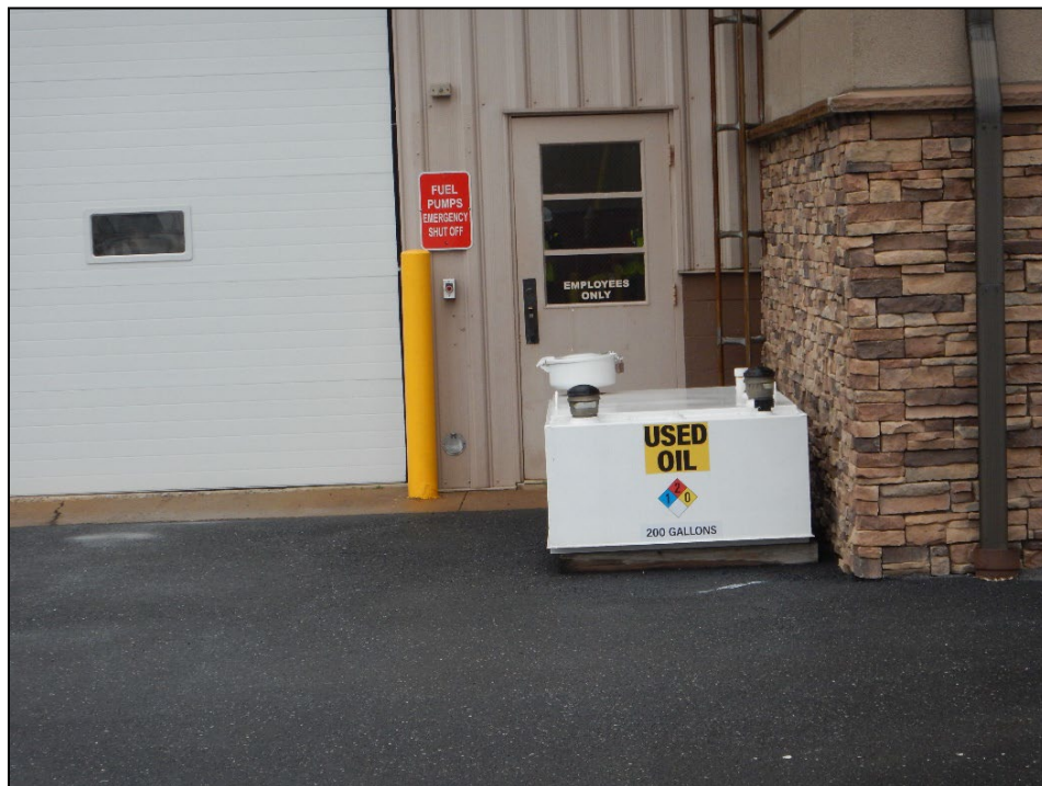
Photograph 8. Township Municipal Building: (DSCN2954.JPG) View, facing north, of the aboveground 200-gallon used oil tank. Township representatives stated that it is double-walled.
