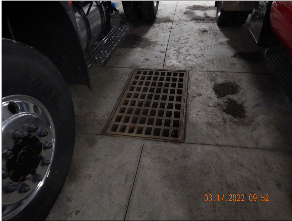
Photograph 13. Township Municipal Building: (DSCN3665.JPG) View of a drain in the second vehicle and equipment storage garage. The drain leads to the oil/water separator before discharging to the sanitary sewer system.
