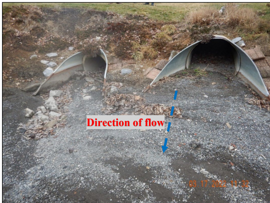
Photograph 40. Outfall #0250 Nicole Drive: (DSCN3717.JPG) View, facing north, of the inlets to the stormwater basin to which Outfall #0250 discharges. Stormwater from Outfall #0250 does not discharge into a surface water.
