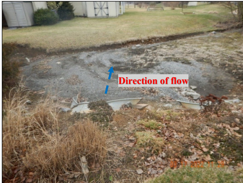
Photograph 39. Outfall #0250 Nicole Drive: (DSCN3714.JPG) View, facing south, of the stormwater basin to which Outfall #0250 discharges (owned and operated by PennDOT).
