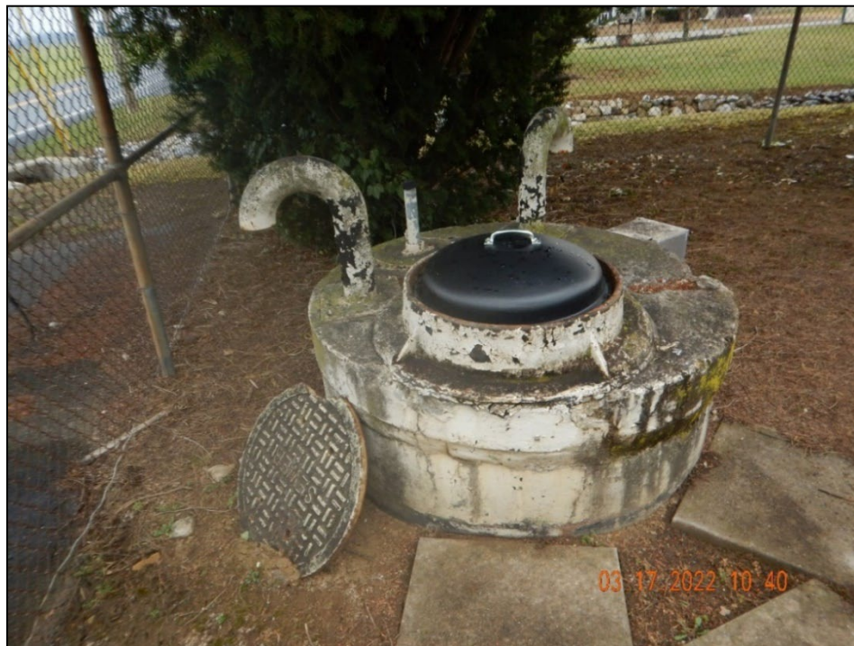
Photograph 30. Lift Station #3: (DSCN3691.JPG) View, facing north, of the Lift Station #3 Grindstone Hill Road (Ryan Lane) Pump Station. The station appeared to be in good condition.
