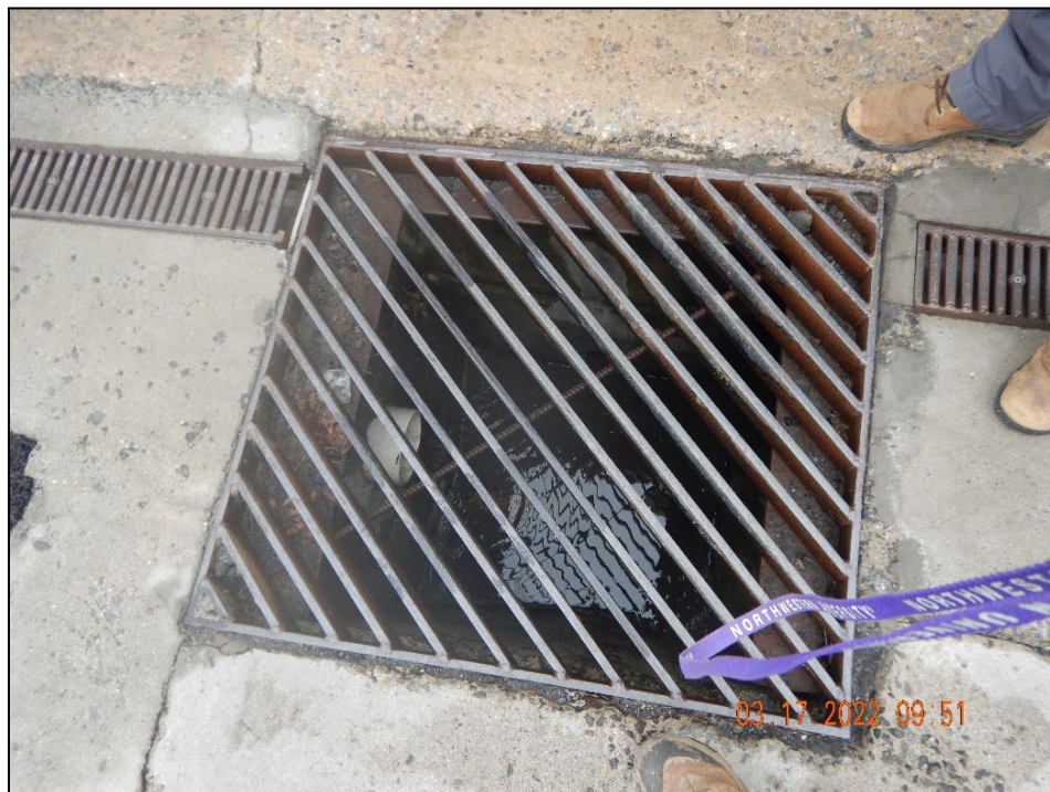
Photograph 18. Township Municipal Building: (DSCN3663.JPG) View inside one of the drains outside of the vehicle storage garages in the Municipal Building.
