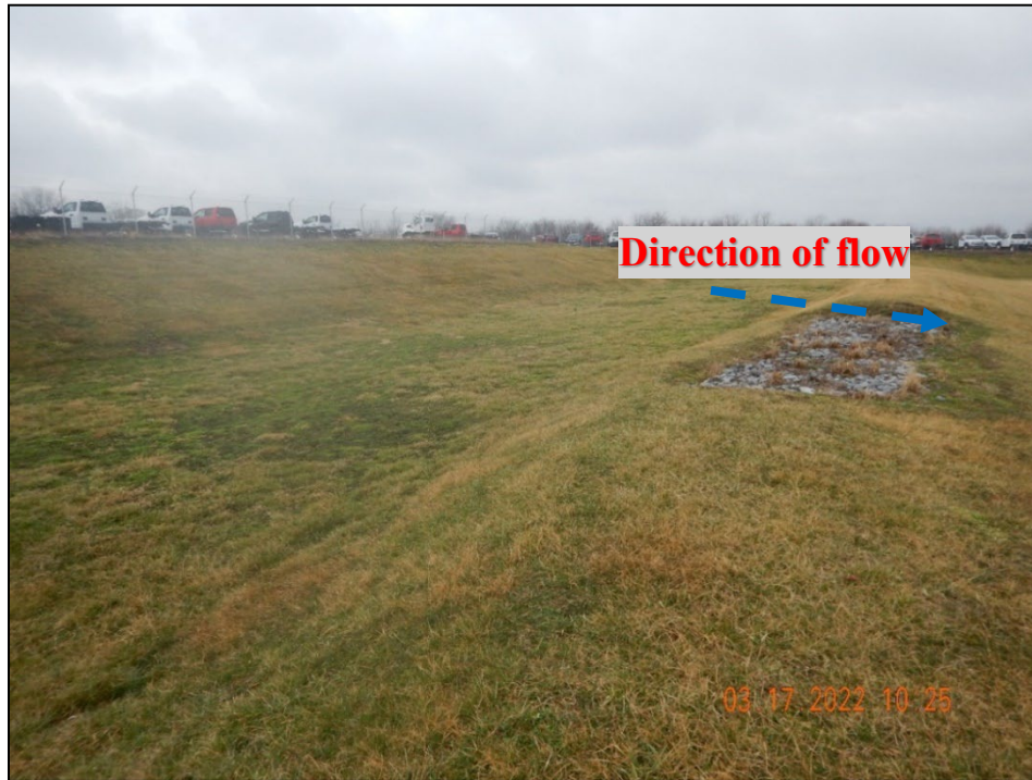
Photograph 25. Vehicle Facility Yard: (DSCN3677.JPG) View, facing northwest, of the second stormwater basin.
