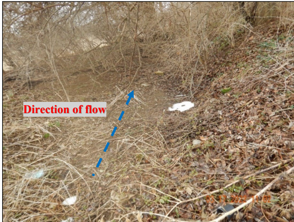
Photograph 35. Outfalls #0240 & #0245 Jason Drive: (DSCN3704.JPG) View, facing south, downgradient of Outfall #0240 of Paddy Run.
