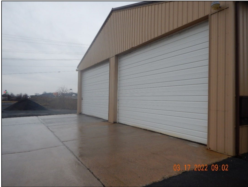
Photograph 1. Township Municipal Building: (DSCN3633.JPG) View, facing west, of the salt and sand storage garage in the Municipal Building.
