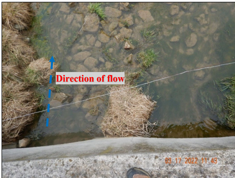
Photograph 42. Outfall #0130 East Weaver Road: (DSCN3723.JPG) View, facing south, downstream of Outfall #0130. The outfall discharges runoff to the unnamed tributary to Conococheague Creek.
