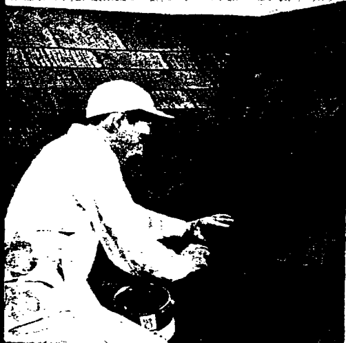
11. Save the roof—now! Nothing about the house is more important to keep in condition than the roof. Small leaks there can become big troubles, in a hurry. When you come to it, reroofing is a job for experts—and your lumber dealer is the man to see. Let him show you the beautiful colors of USG* Thick Butt asphalt shingles, such as Venetian Red, shown here. At the same time, keep your gutters and downspouts in good repair. Winter's ahead!
