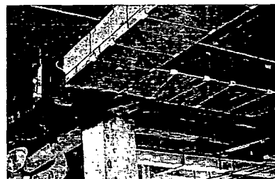
For Ducts. Light-weight blocks of FOAMGLAS were easily applied to these metal air conditioning ducts at the Moses H. Cone Memorial Hospital, Greensboro, North Carolina.
