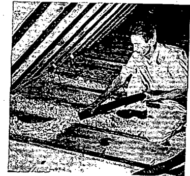
The blowing method is used in existing houses between walls or floors
