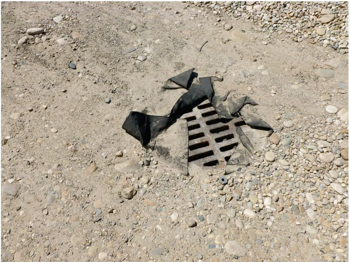
Photo 9 / P1000883 – Storm Drain, to catch basin
