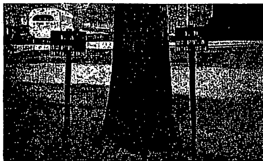
OUTDOOR VALVE markers give compass bearing and distance so personnel can easily locate valve. Sign also identifies valve
