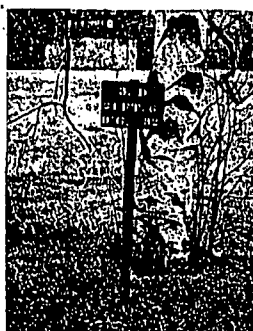
OUTDOOR VALVE markers give compass bearing and distance so personnel can easily locate valve. Sign also identifies valve
