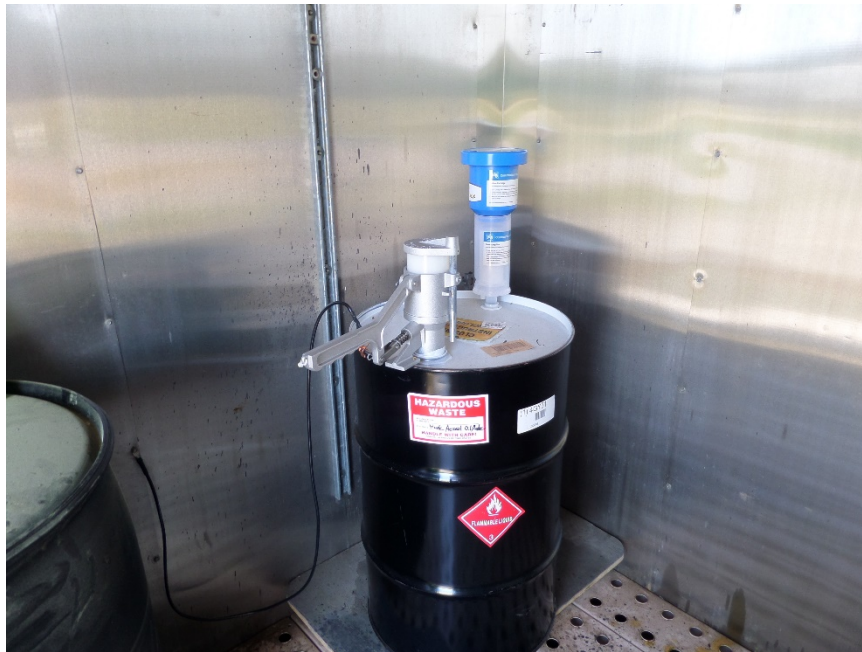
Photograph 7: Shelter A – Hazardous waste accumulation container with aerosol can puncturing device to empty hazardous waste aerosol oil/lube cans generated at the facility.
