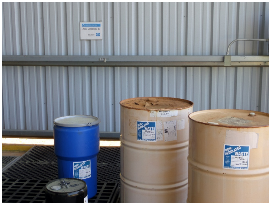
Photograph 2: Non-RCRA regulated grease waste containers in the facility's hazardous waste central accumulation area.
