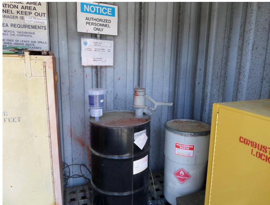
Photograph 15: Munitions Storage Area – In SAA 012, the inspectors observed one 30-gallon hazardous waste container with an aerosol can puncturer attached to the container's bung and one 14-gallon hazardous waste paint waste container.
