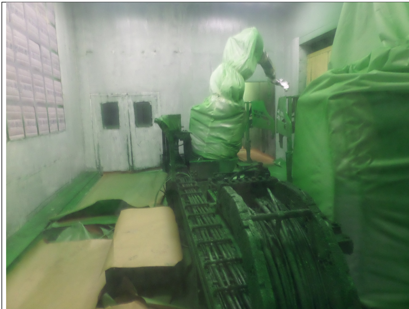
Wilbert. Paint Department. Robotic Primer Paint Booth. Observed container not labeled with the words hazardous waste and no hazard indicator. Photograph 4 taken at 11:07 a.m.
