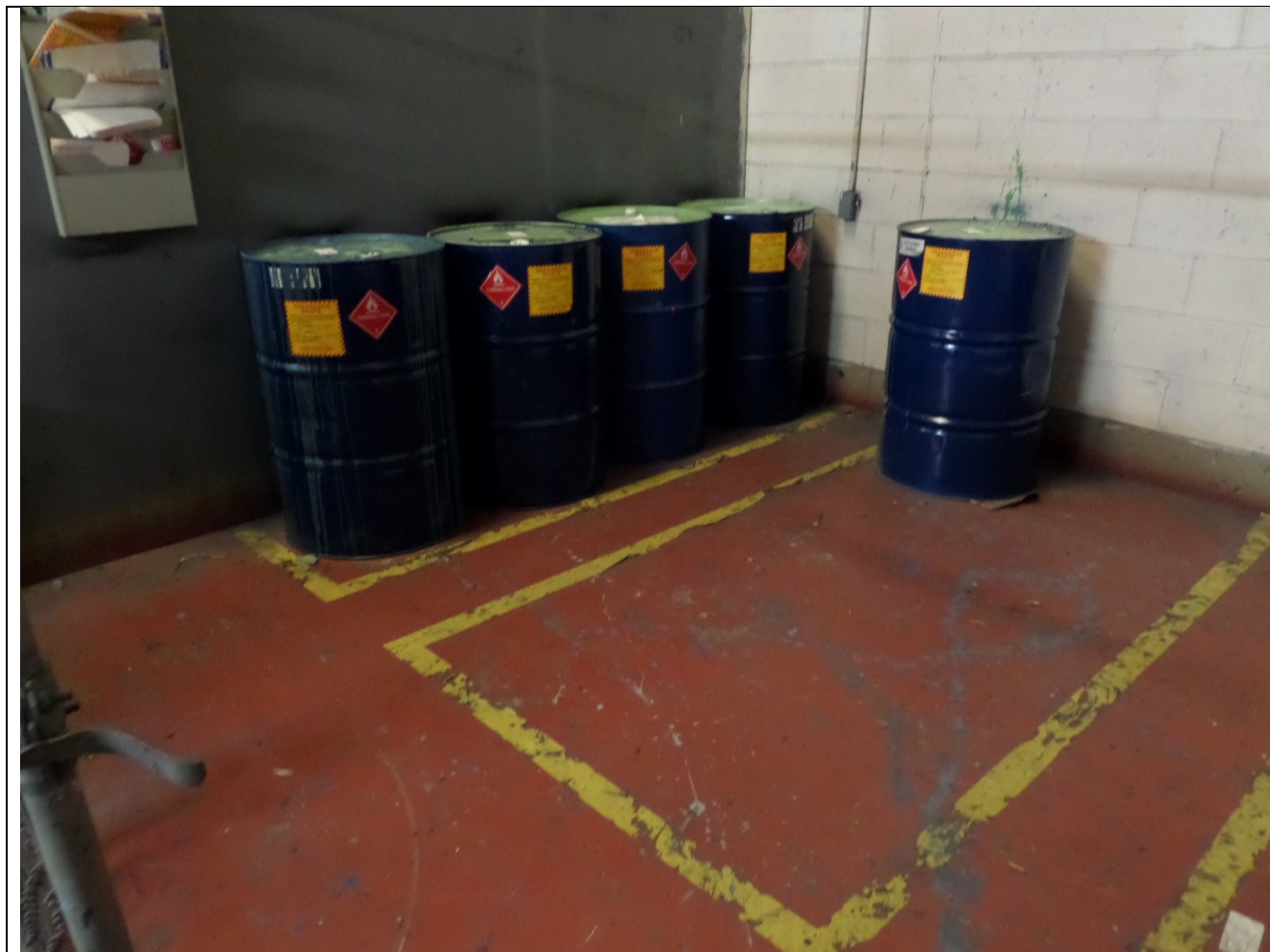
Wilbert. CAA/90-Day or Less Accumulation Area. Observed containers accumulating hazardous waste. Observed the floor epoxy appeared to be deteriorating. Photograph 8 taken at 11:39 a.m.
