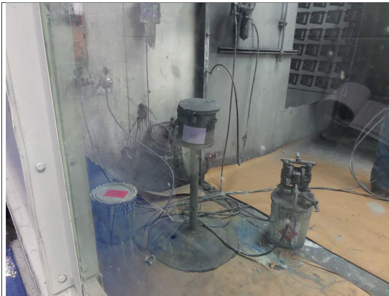
Wilbert. Paint Department. Manual Paint Booth 4. Observed a container was not marked/labeled with the words hazardous waste and no hazard indicator. Photograph 12 taken at 11:55 a.m.
