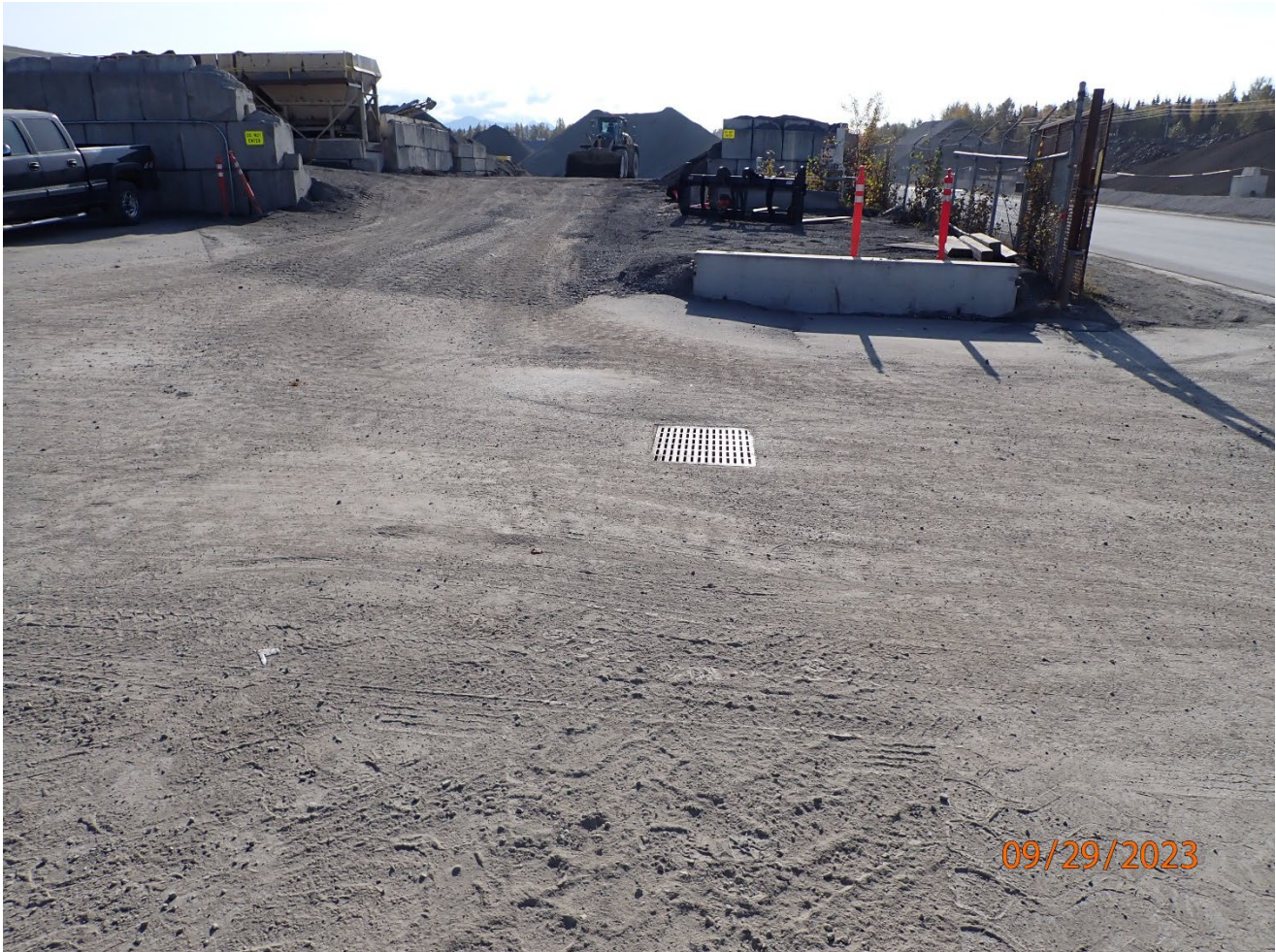
Photo 1 - Storm drain that leads to water pump
