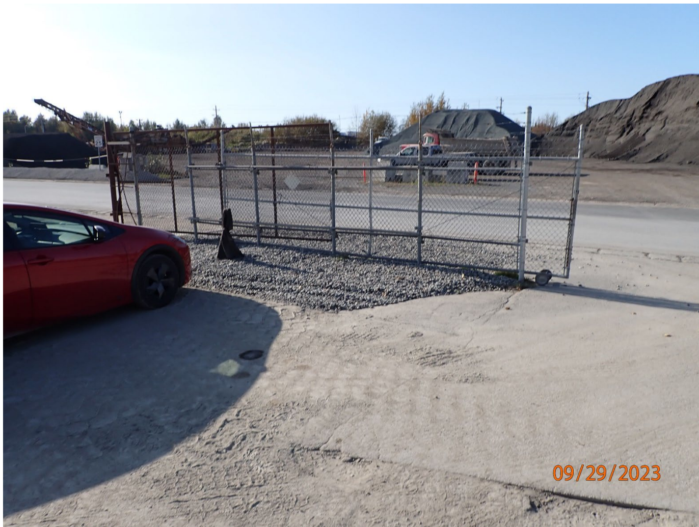
Photo 4 - Rock outfall with sock filter over pipe
