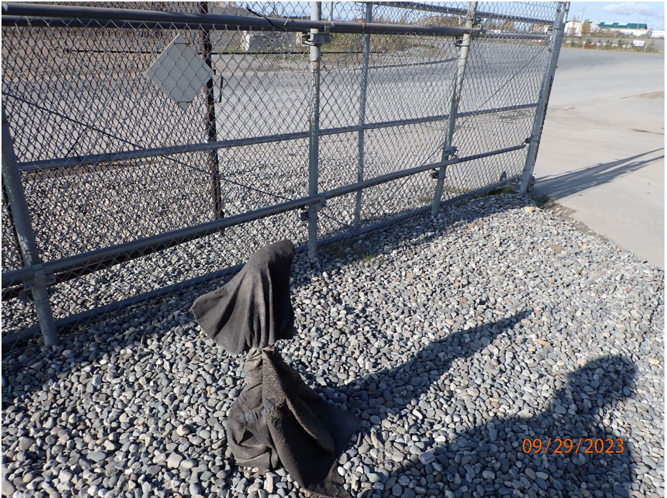
Photo 3 - Rock outfall with sock filter over pipe
